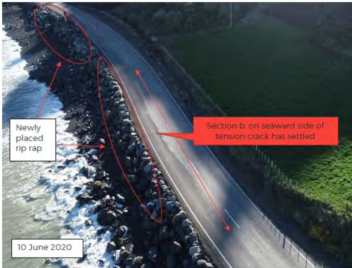
Figure 32: Drone imagery in central section of Section 1 from May and June 2020, showing crack and displacement of carriageway in foreground and earthworks to lower road level in middle distance. Newly placed rip rap indicated.
