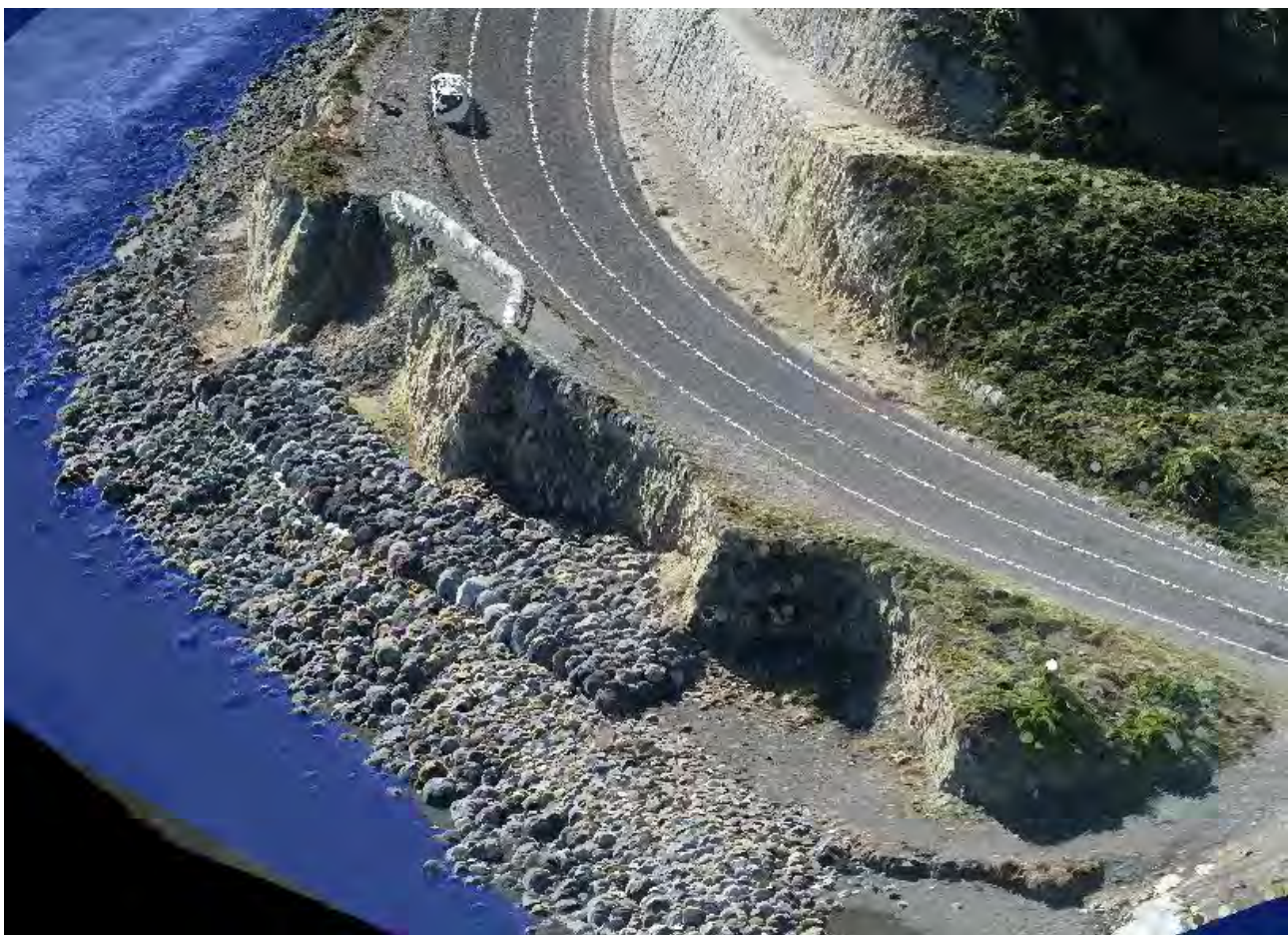
Figure 37. Screenshot from 3D model showing S4.4 eroded areas and placed rock rip-rap, which are currently creating alongshore irregularities.
