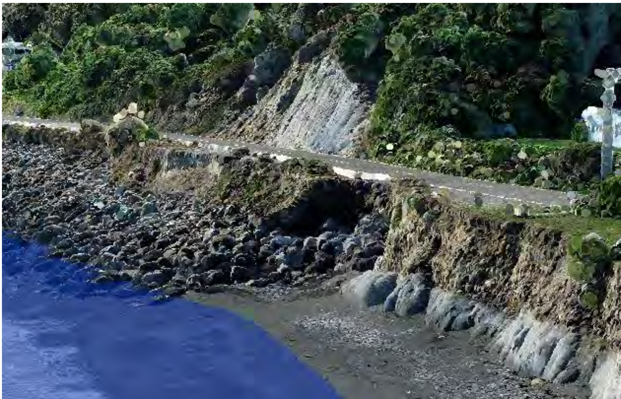
Figure 35. Screenshot from WSP's UAV model, showing the significant dropout in Section 3.4.
