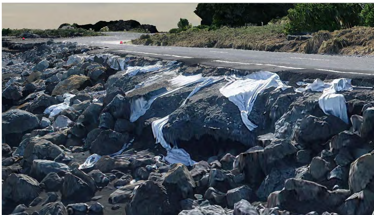
Figure 30: Section where stabilising cement has been used in the road sub-base in the northern section of the DOC Station reach.
