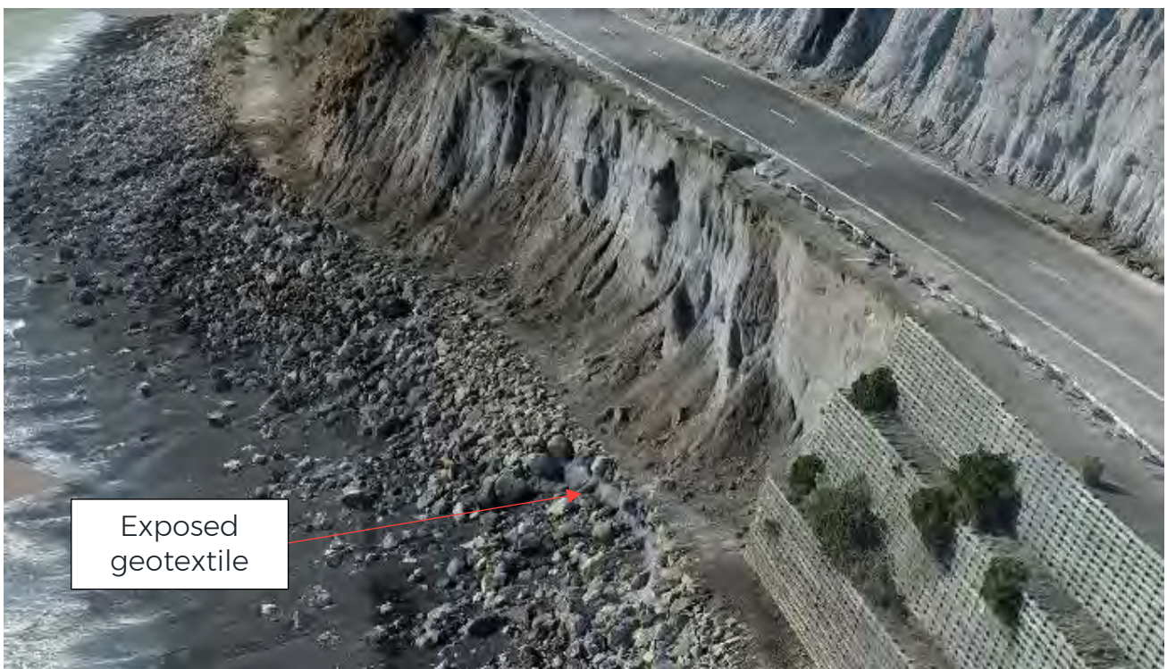
Figure 40: Sections of exposed geotextile at Whatarangi Bluff, where the rip rap structure has collapsed and needs repairing or replacing to reinstate effective coastal protection. [top] South of concrete wall (CONC2 in the preliminary risk assessment table). [bottom] North of crib wall (CRIB1).
