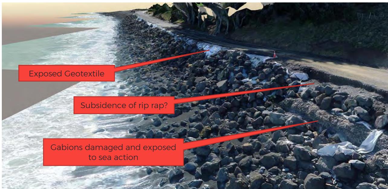
Figure 29: Coastal protection structures in Section 1.1. From WSP's UAV model, May 2020.
