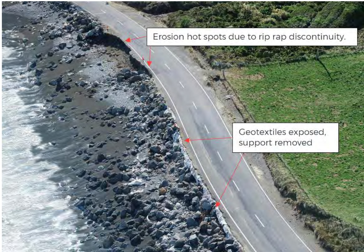
Figure 31: Screenshot of Section 1, DOC Station, showing from aerial view erosion hot spots and exposed geotextile at the road edge.
