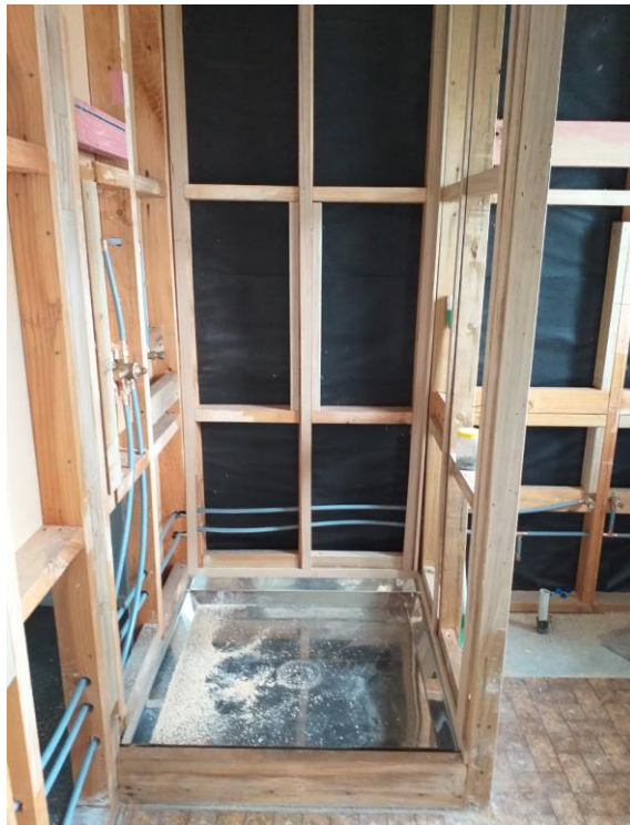
Bathroom during upgrade/repairs
