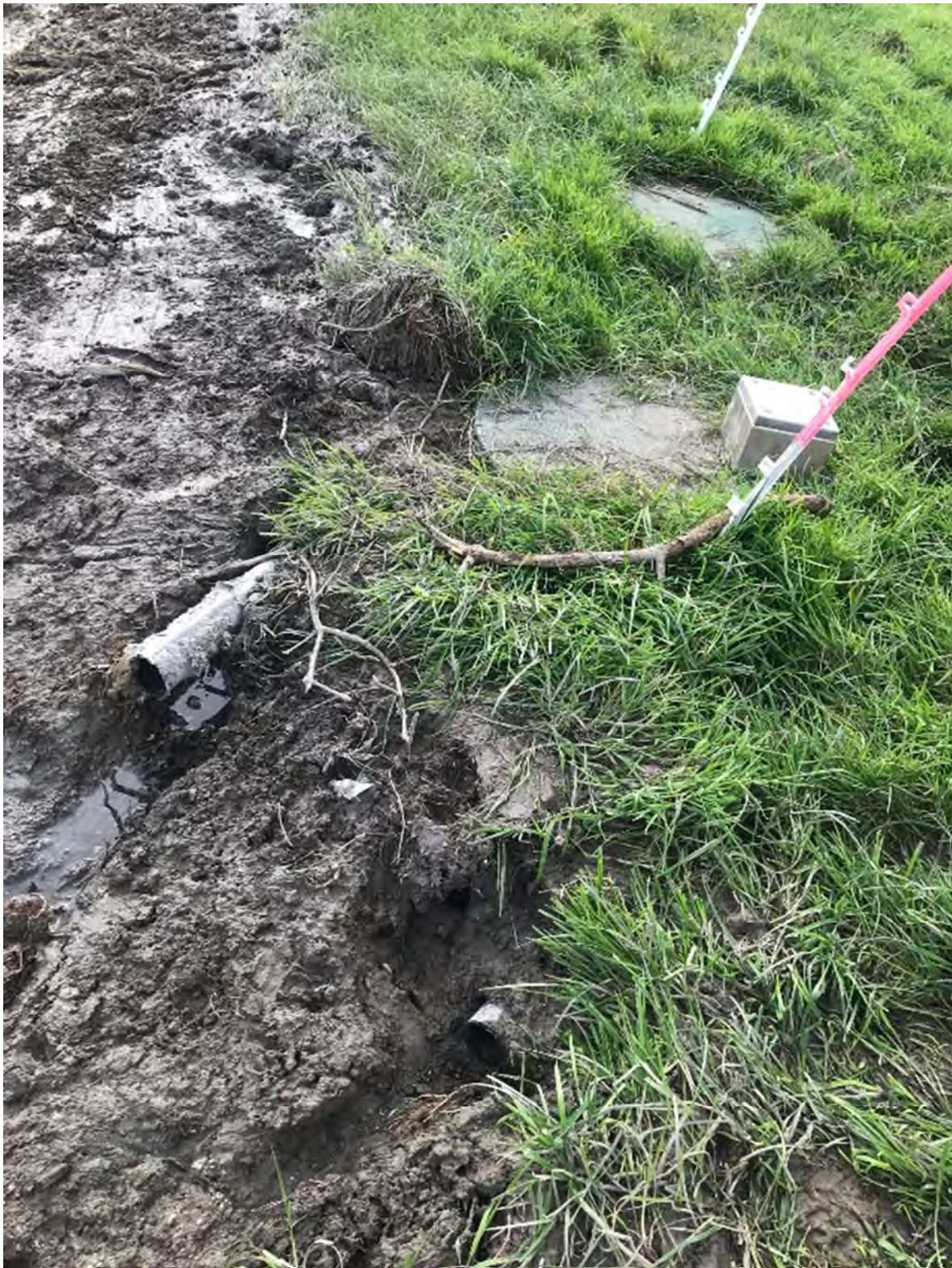
Figure 1: Severed Main Pipe
