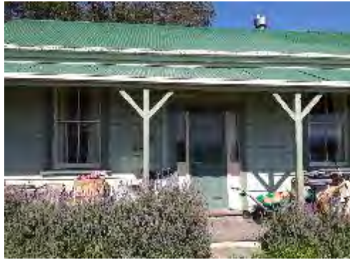
Pain Farm Cottage Exterior Before
