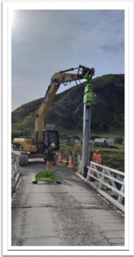
Pile driving Tora farm Settlement bridge.
