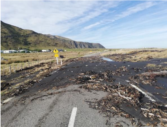
Cape Palliser Rd tidal swell damage
