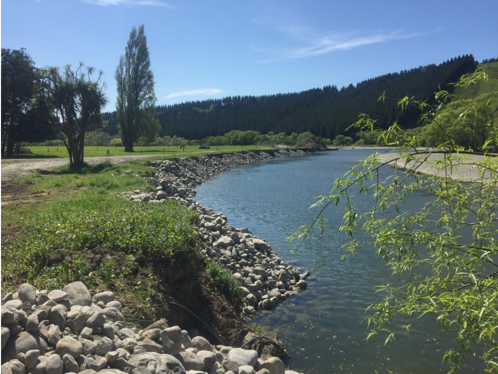
Huangarua River Left Bank Flood Damage Repairs
