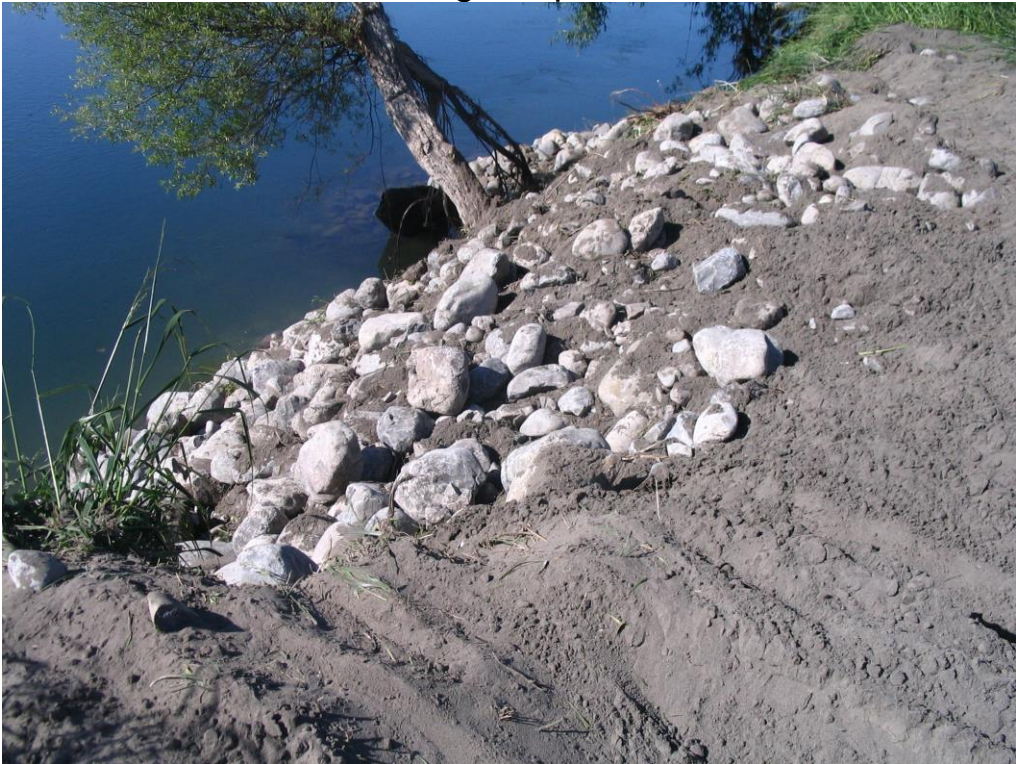
Tucker’s Bank Flood Damage Repairs
