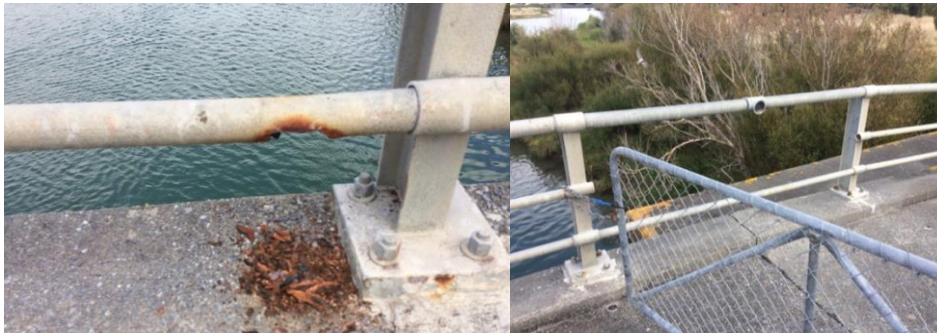
Figure 3 Barrage Gates Safety Railings
