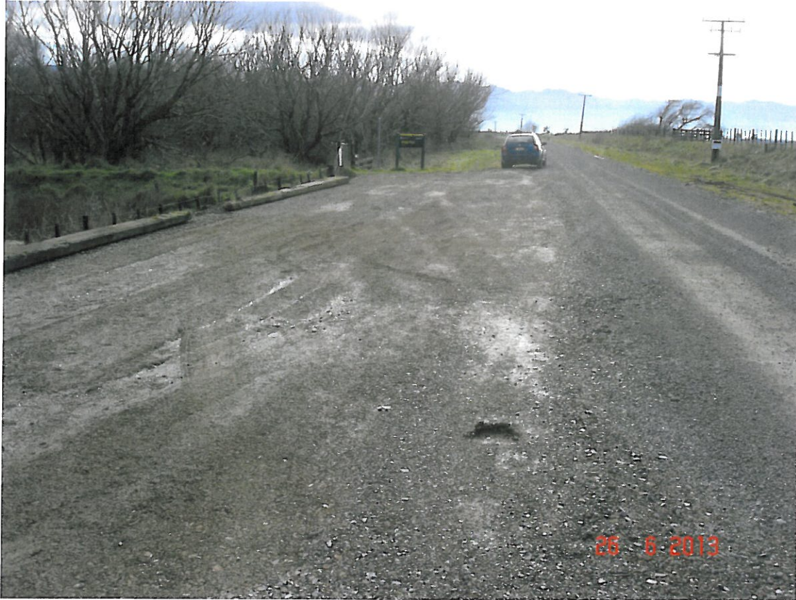
Recently constructed car park at Boggy Pond
