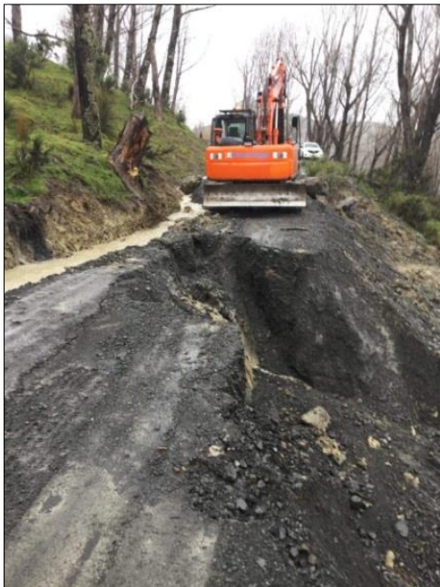
Drop out and road closure at Ushers Hill, White Rock Road
