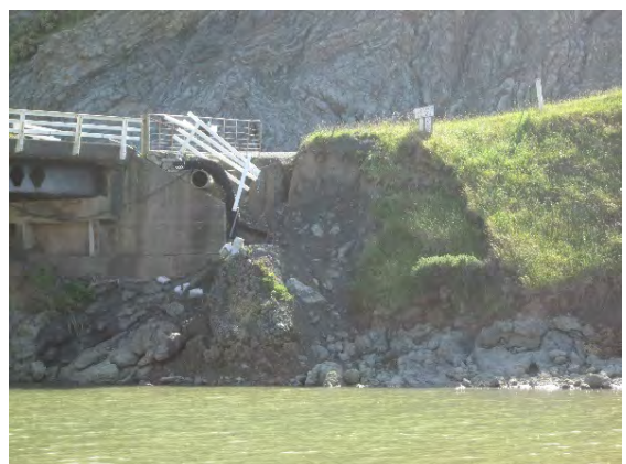
Te Awaiti Bridge abutment washout
