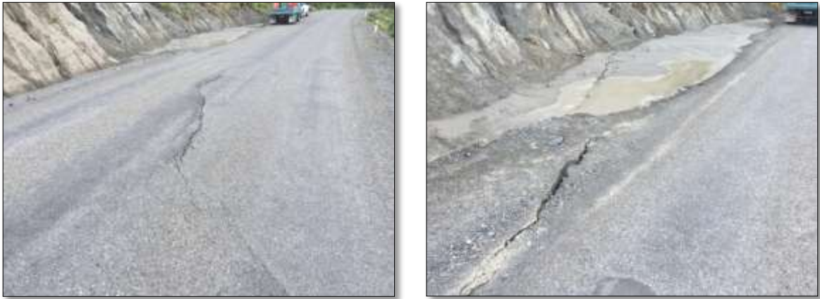
Fig 6.2.b: Photos following the earthquake event
