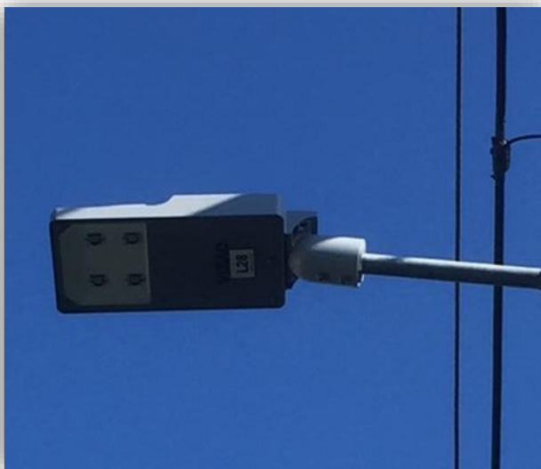
New LED light installed
