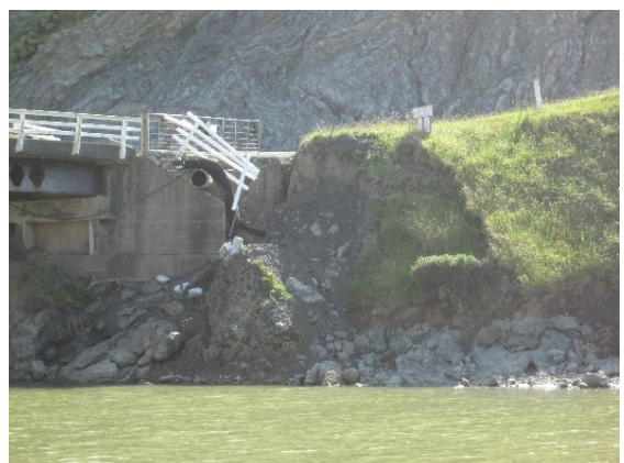
Te Awaiti Bridge abutment washout
