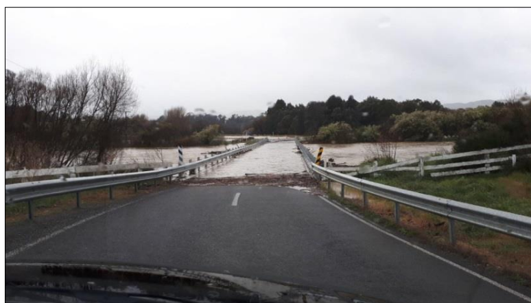
Flooding and road closure at Haungarua Bridge, Ponatahi Road
