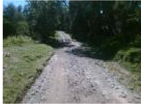
Glendrynoch Rd bridge approaches
