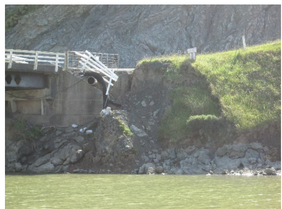
Te Awaiti Bridge abutment washout
