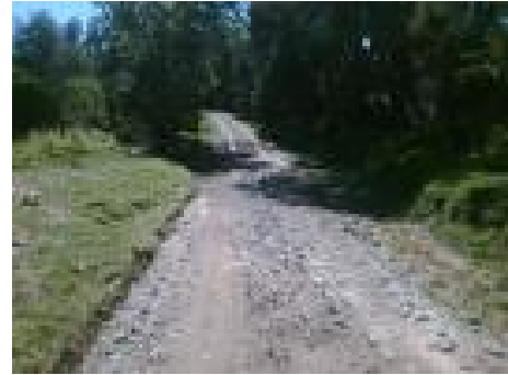
Glendrynoch Rd bridge approaches
