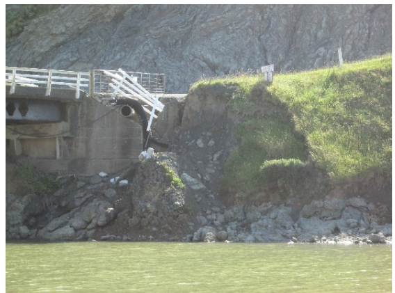
Te Awaiti Bridge abutment washout
