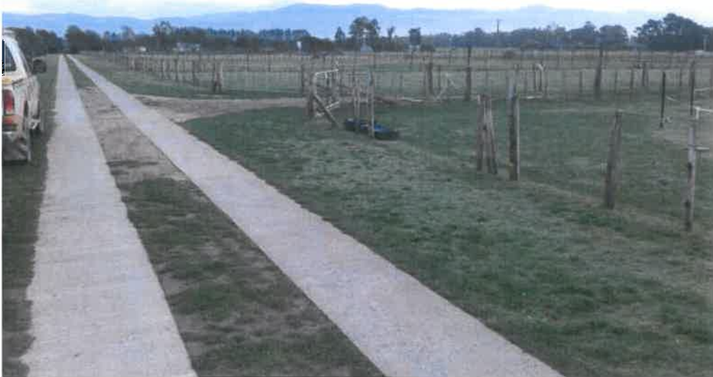
Photograph 3: Concrete drive within Lot 3 to the dwelling
