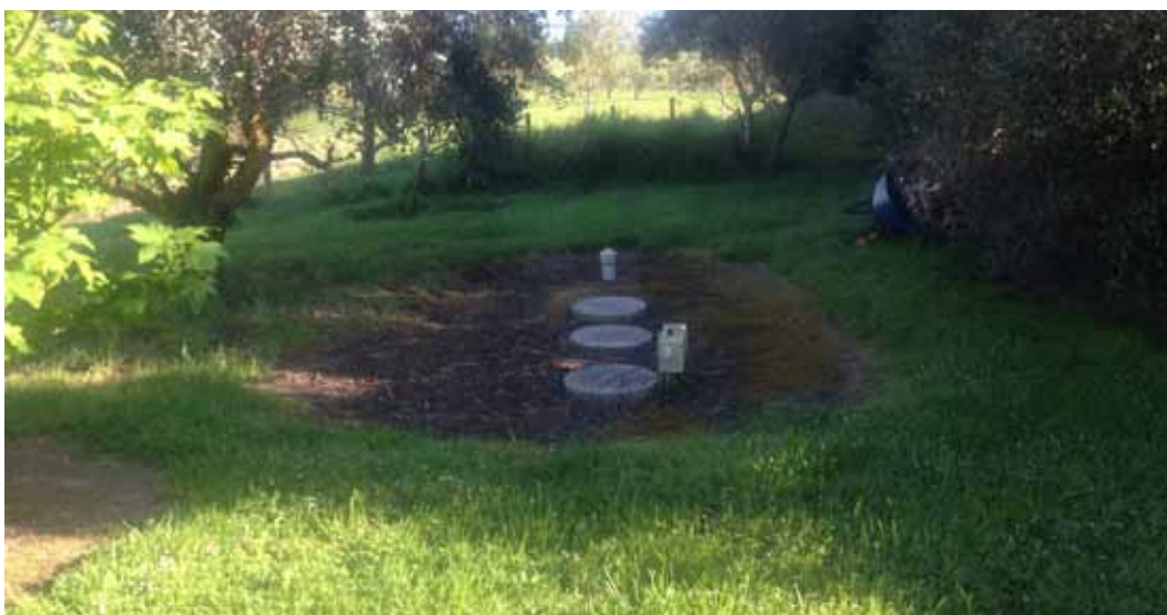
Photograph 4: Effluent disposal system within Lot 2
