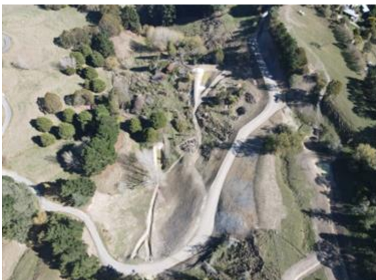
Pictured: Hinekura earthworks, January 2024.
