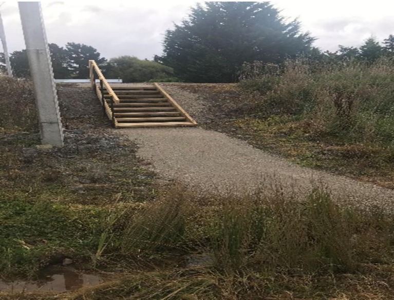
Above: The new access steps for the Pirinoa Water Treatment Plant
