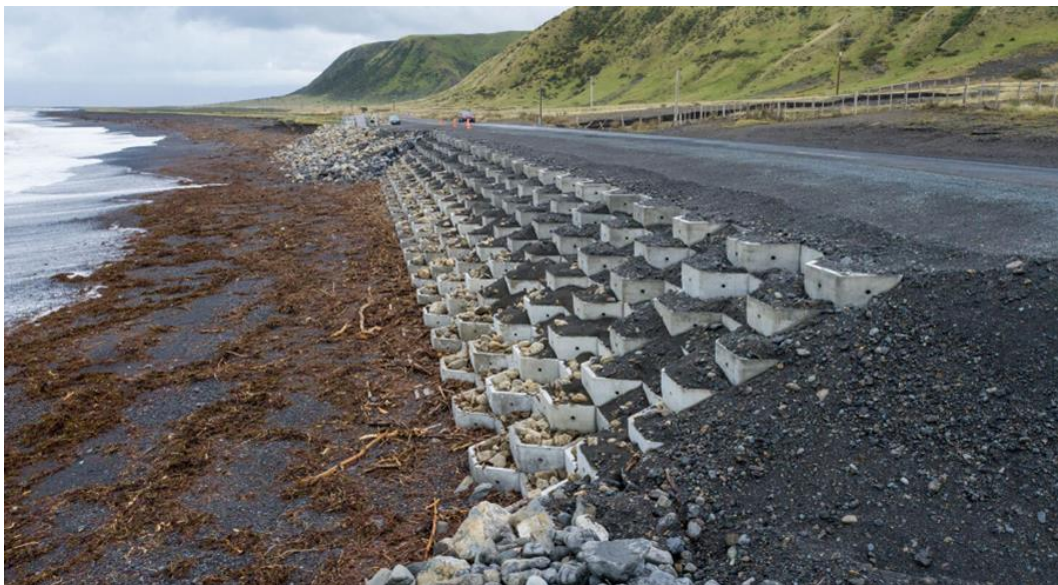
Pictured: Cape Palliser Road remediation – before, during and after.
