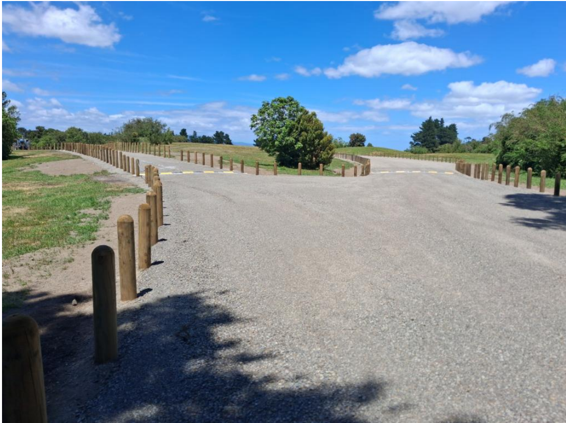
Figure 2 Resurfaced Otauirā Reserve carpark
