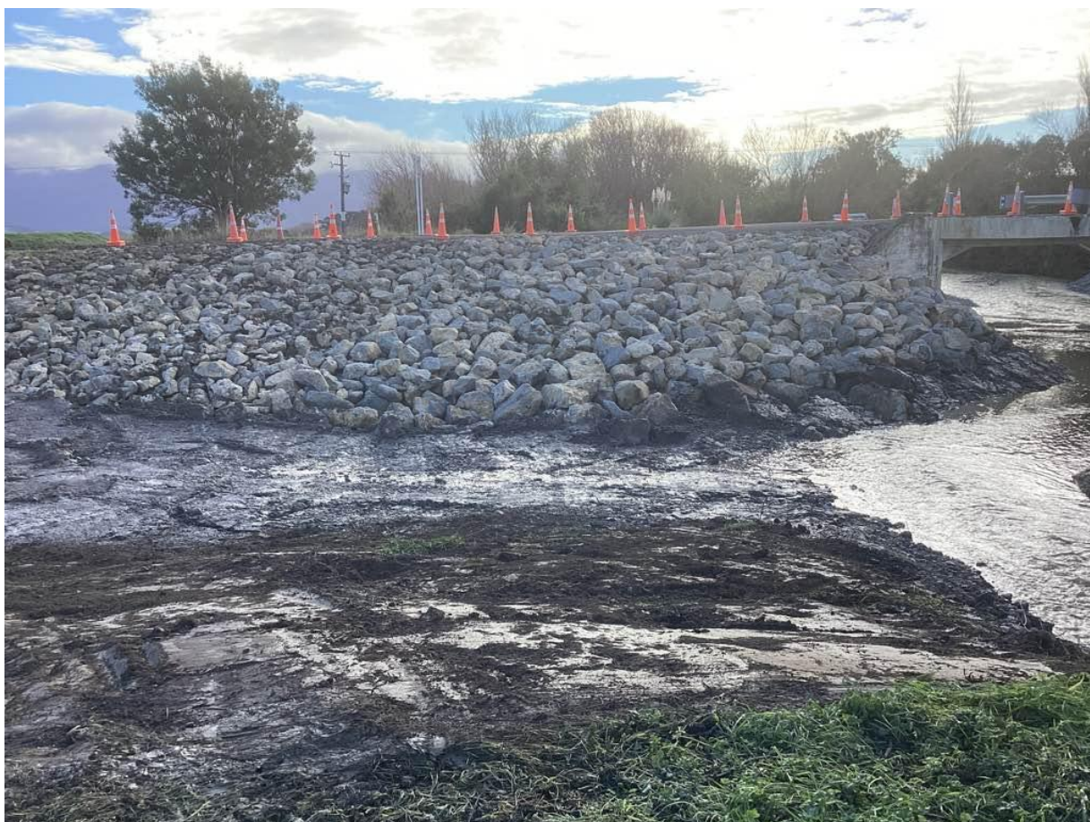
Figure 6 South end of Tūranganui bridge remediation following February severe weather
