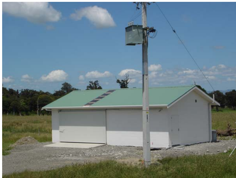
New wastewater building in Featherston
