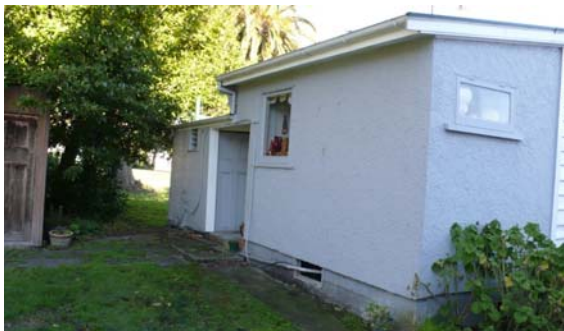
Northeast corner where the lean-to has been stucco clad
