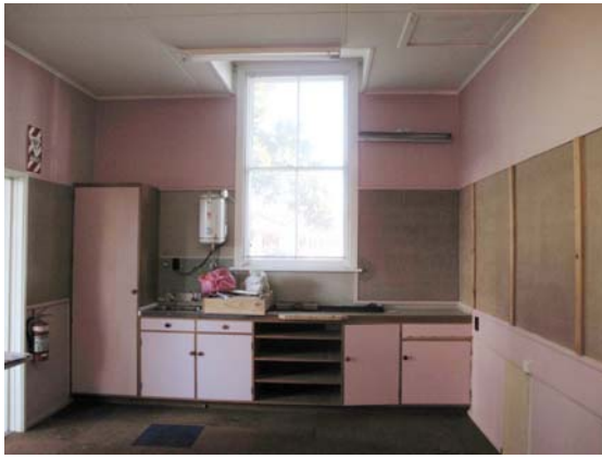
Kitchen – New lowered ceiling boxed around original high front wall window
