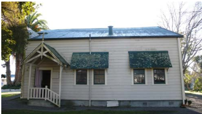
South wall, with mould and lichen growth, broken sub-floor access door.
