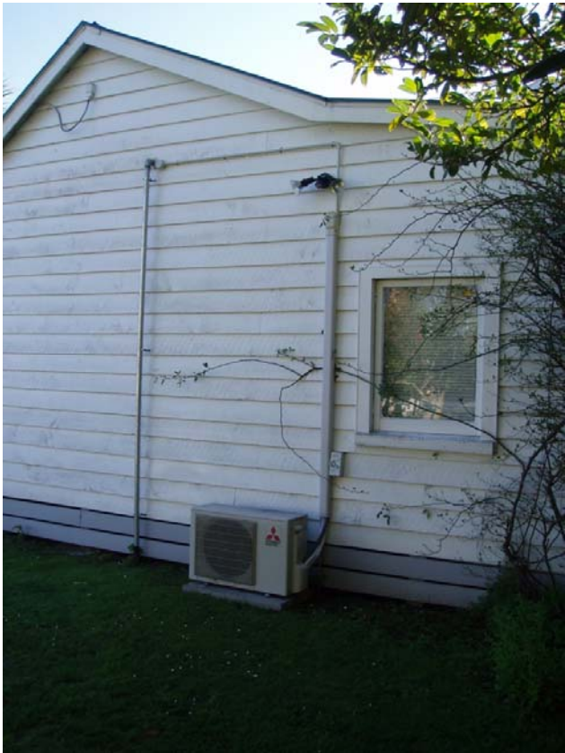
South Elevation– Unpainted sprinkler pipe. Wall needs cladding
