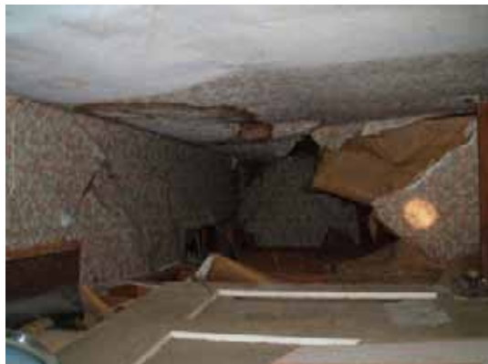
Original wallpaper exposed between new and original ceilings
