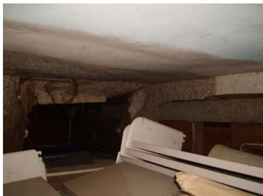
Space between new lower ceiling and original with stored stuff.
