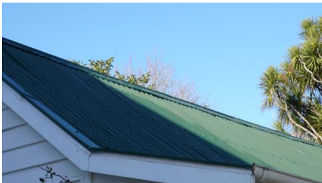
Roofing with some loose ridging
