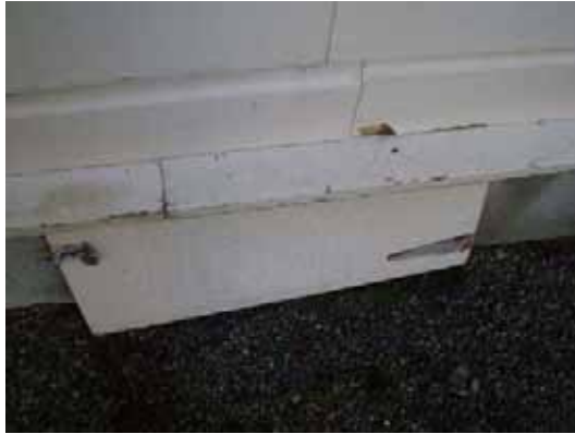
Sub-floor access door with broken hinge
