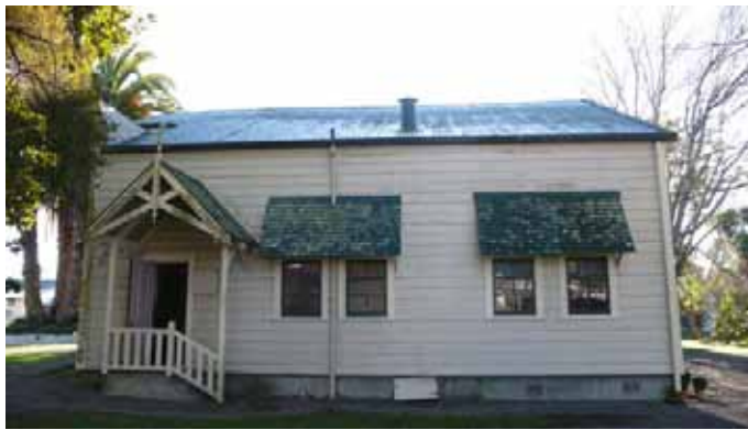
South wall with added "timber gothic" styled porch and window hoods
