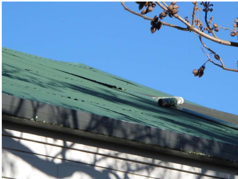
Roof, showing loose roofing sheet. (and (disgusting) downpipe detail)
