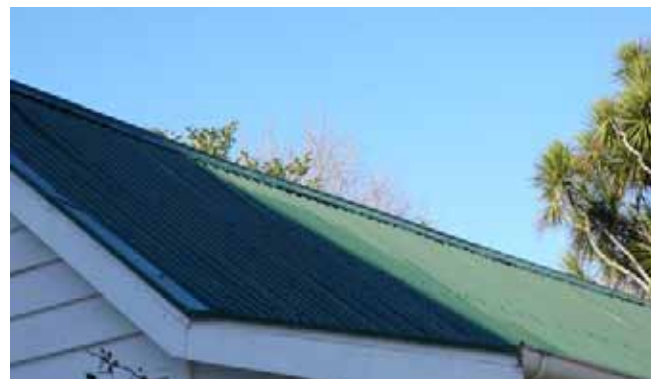
Roofing with some loose ridging.
