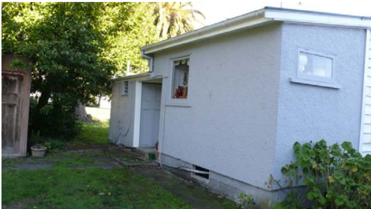
Northeast corner showing the stucco clad lean-to and the roof step which is oddly placed over the porch.
