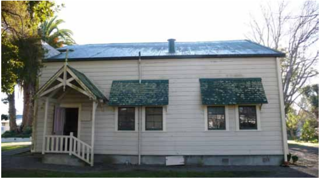
South wall, with mould and lichen growth, broken sub-floor access door.
