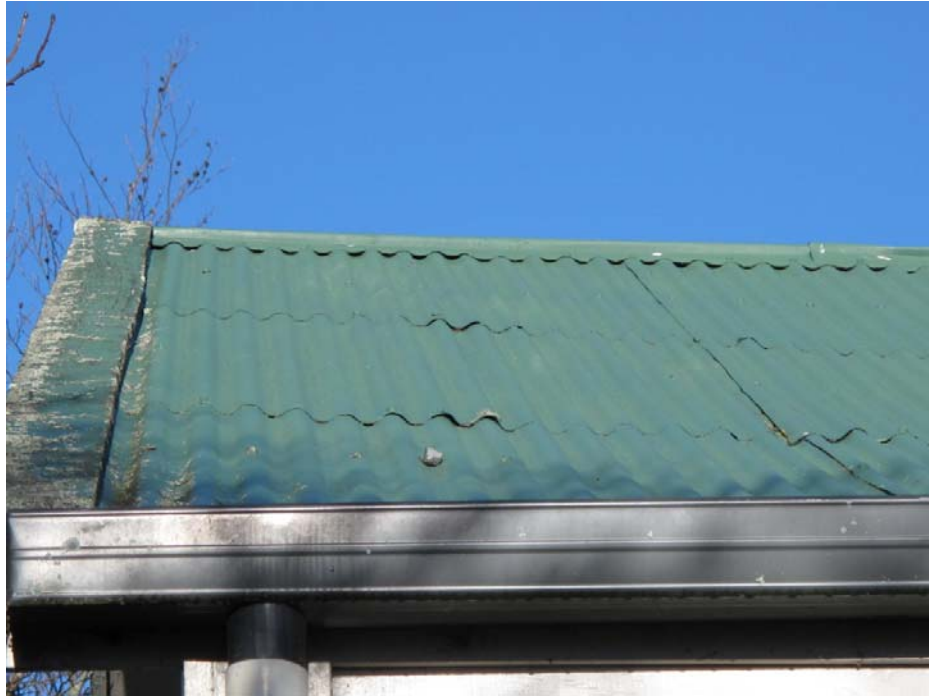
Roof, showing sheet overlaps, ridging and timber rear barge capping.
