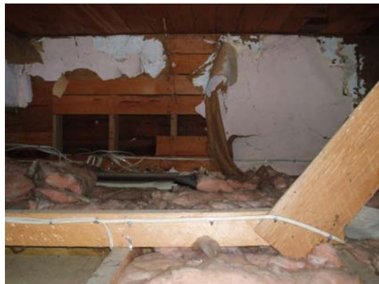
Space between new and original ceilings, showing original wallpaper on scrim and sarking
