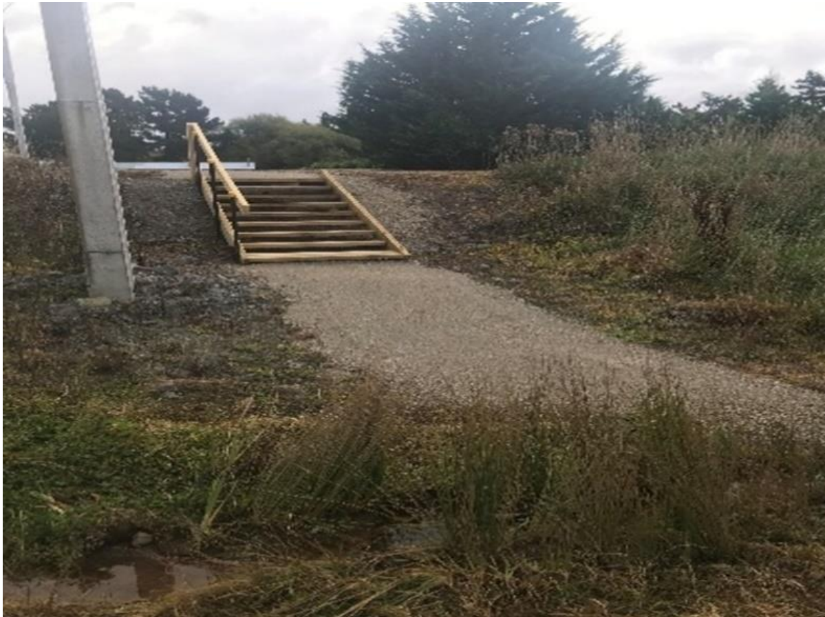
Above: The new access steps for the Pirinoa Water Treatment Plant
