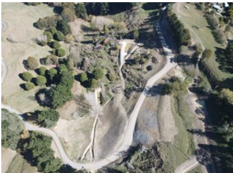
Pictured: Hinekura earthworks, January 2024.
