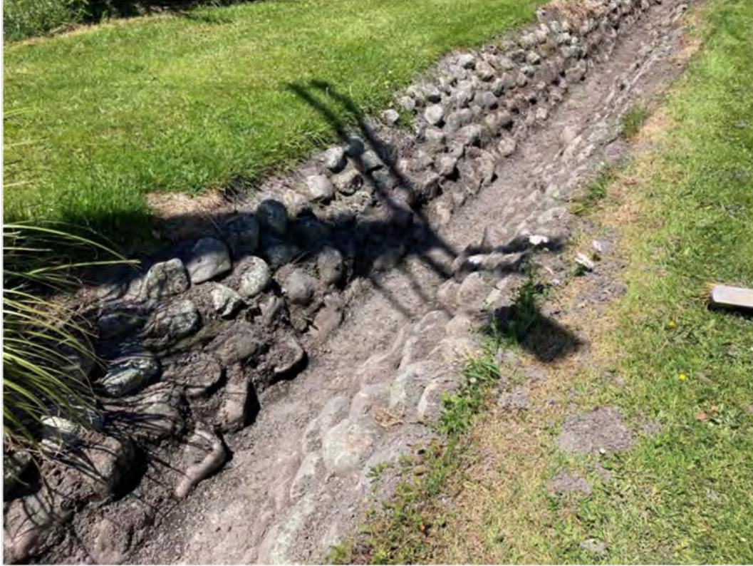
Drain cleaning alongside footpath to Featherston Railway Entrance
