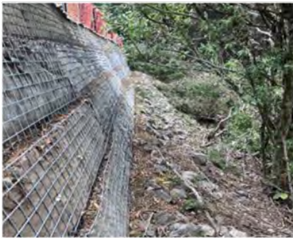
Site 1 works completed
