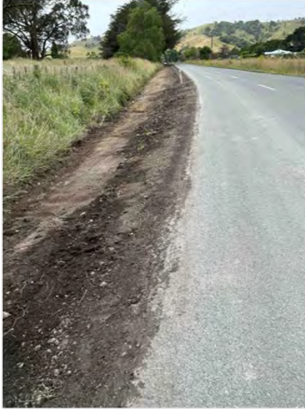
Drain cleaning on Longbush Road
