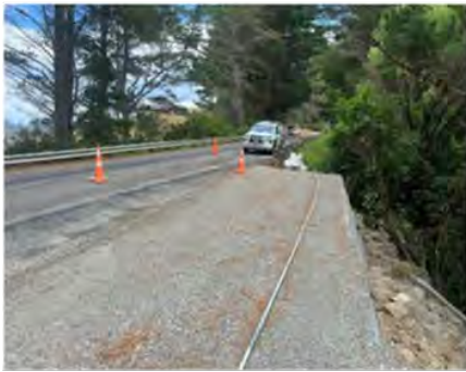
Site 2 works completed
