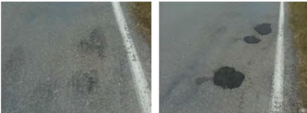
Pothole repaired on Ponatahi Road
