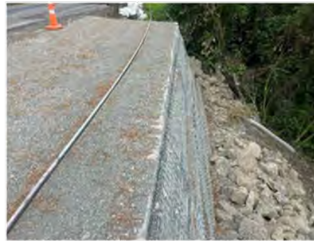
Site 2 works completed
