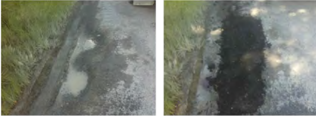
Edge break repairs on White Rock Road
