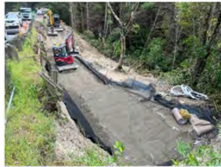
Site 3 works commenced and in progress
