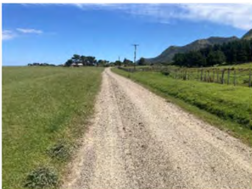
Unsealed road grading and metalling on Pahaoa Road
