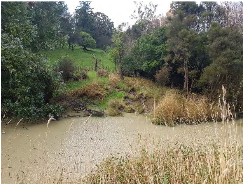
Fissure (western landslide margin) going upslope of dam
