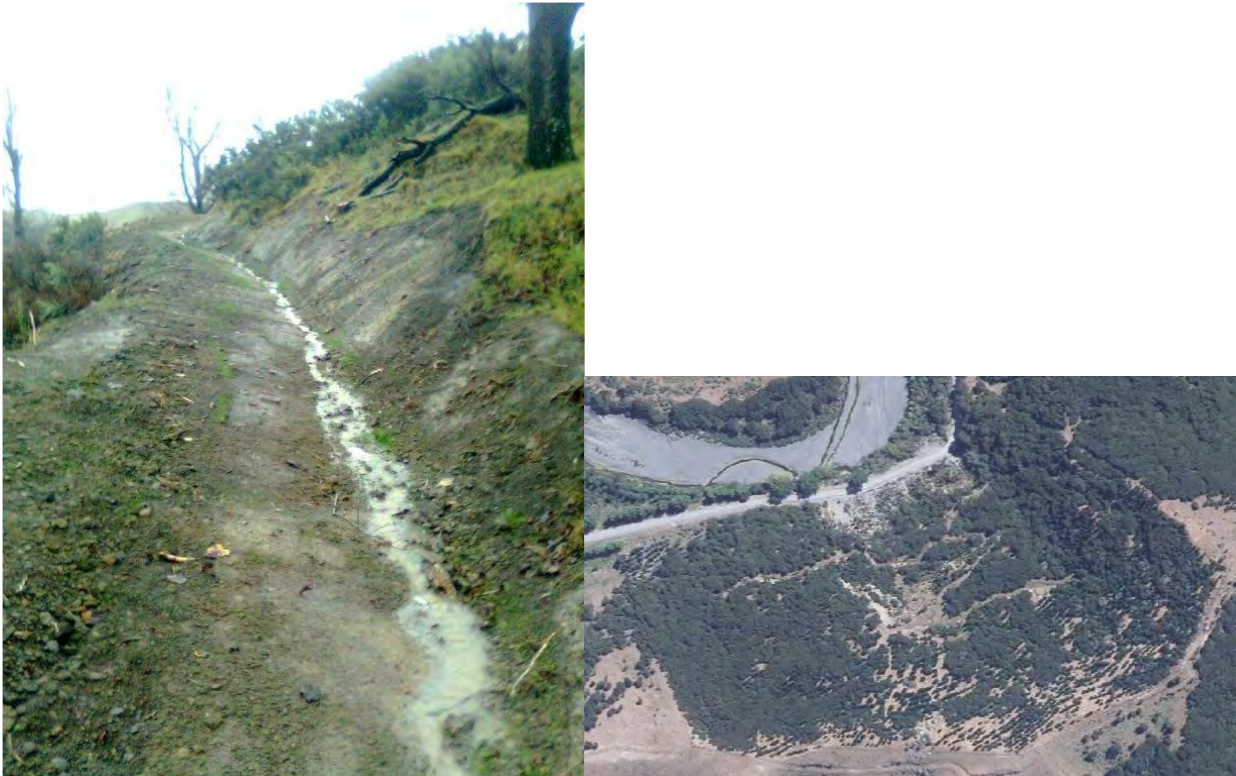
Picture of a v drain, with the aerial view of this v-drain on the right, White Rock Road.
