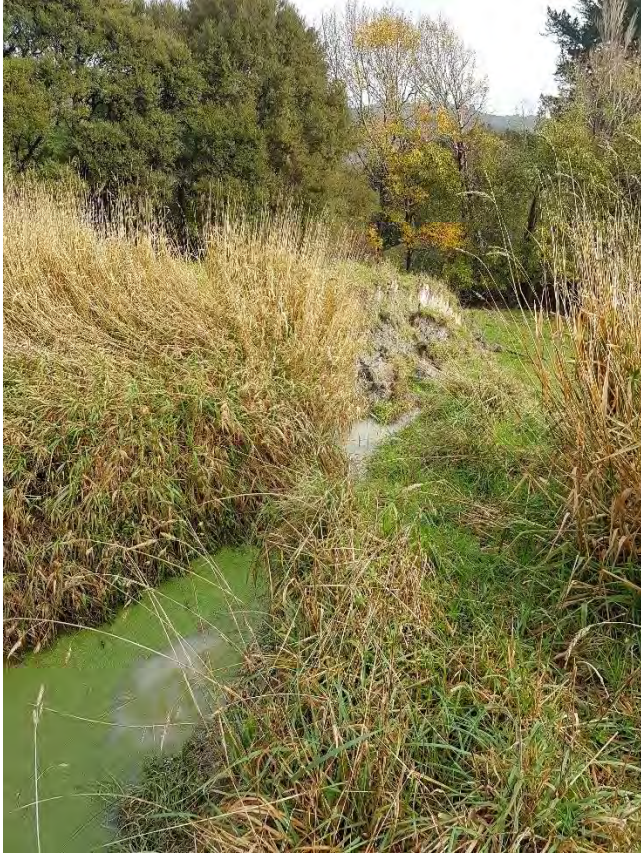
Water breaching dam along line of fissure (moderate flow) view downslope
