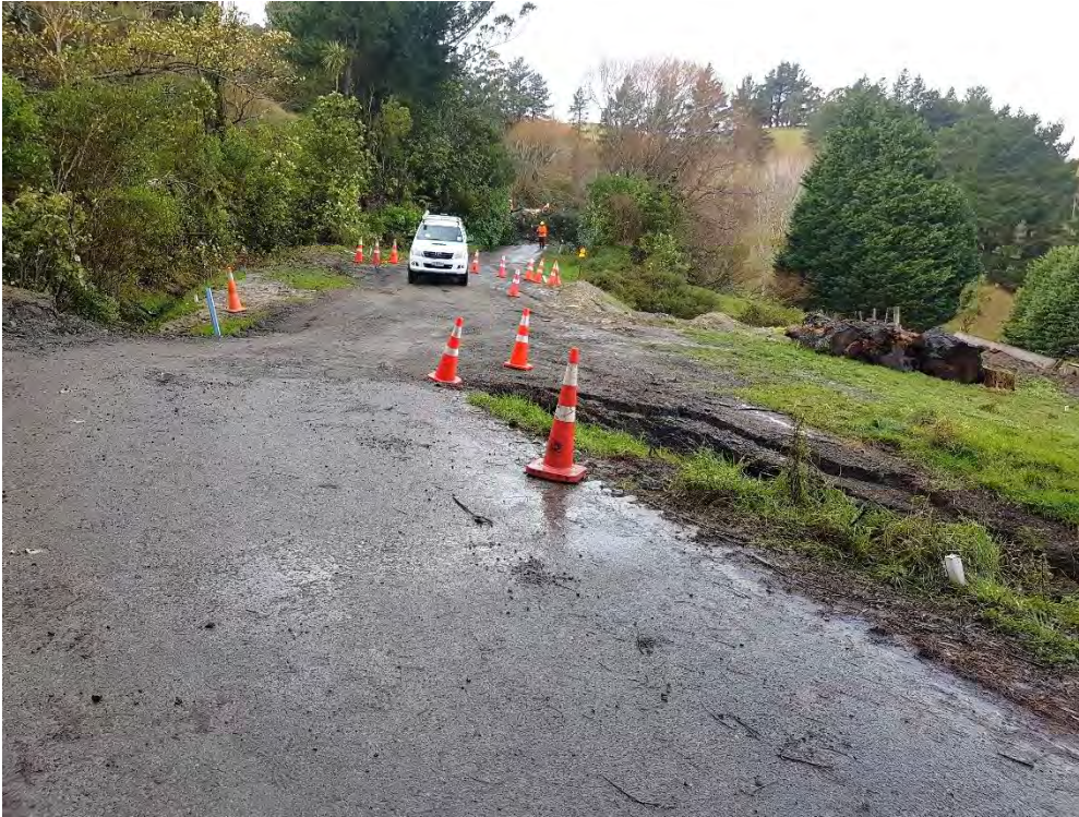
Photo 1: Site on 29 June 2021, showing translation of the road downslope. Lateral scarp in foreground has been removed to allow arborists in to cut down tilting trees (arborist staff visible in background). White SWDC monitoring pegs visible at right and just to left of blue culvert marker.
