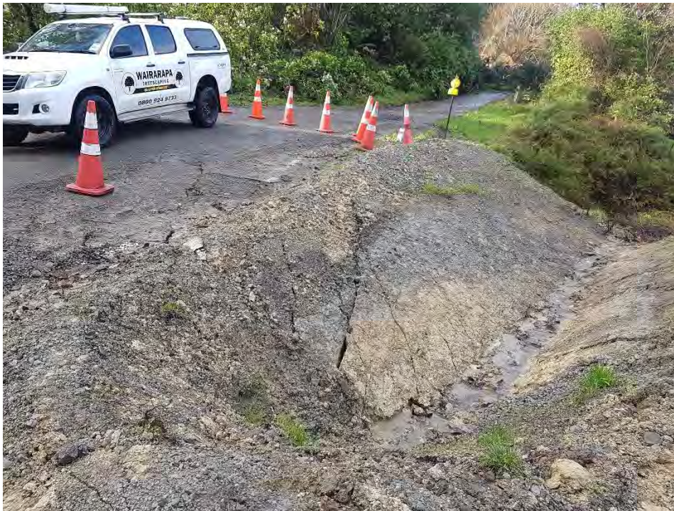
Sharp tension cracks in (1 year old) drain
