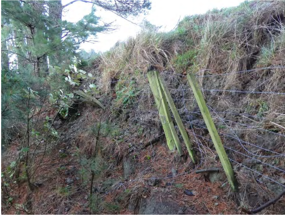
Bulging at eastern margin of landslide has just reached fence (and trees)
