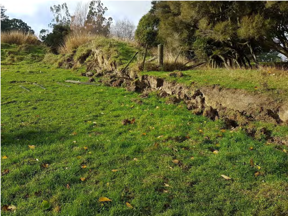
Landslide margin through/ below dam face
