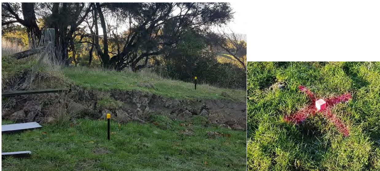
Photo 2: Waratah extensometer below dam (offset broken fence at left) and Photo 3: Survey peg
