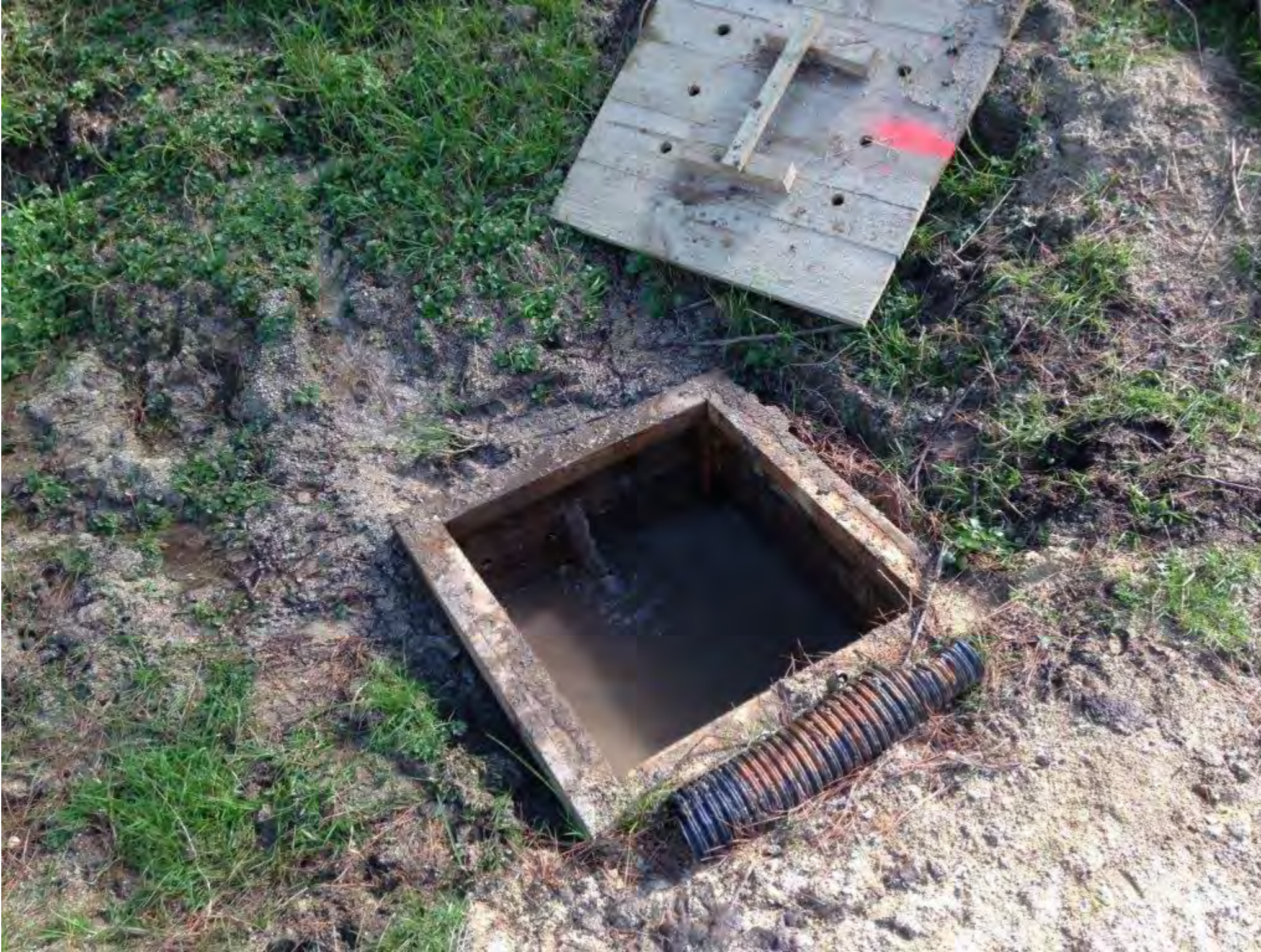
Picture of a catching box, with inlet visible where water is running. An outlet is on the other side of the box.
