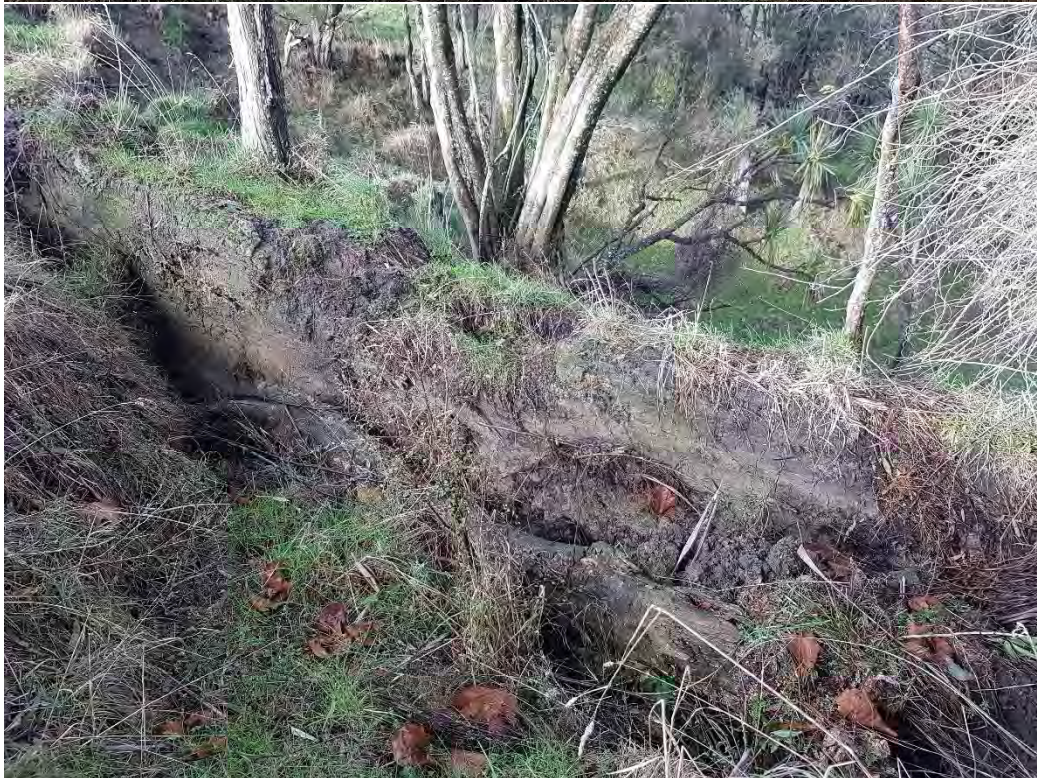
Eastern margin of landslide pushing steeper slopes below and causing secondary movement onto steeper slopes above road. Subhorizontal striae visible on both photos showing main movement is very low angle (near horizontal).
