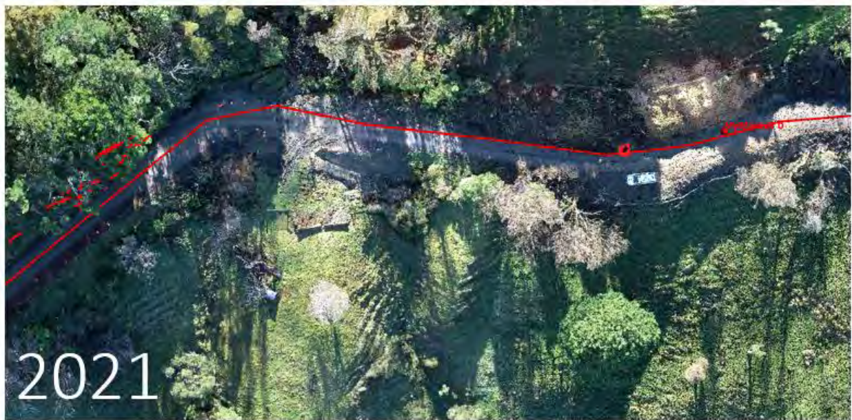
Figure 3: Movement of the road from June 2020 to July 2021. Red line remains in the same location showing the movement of the road from north to south.
