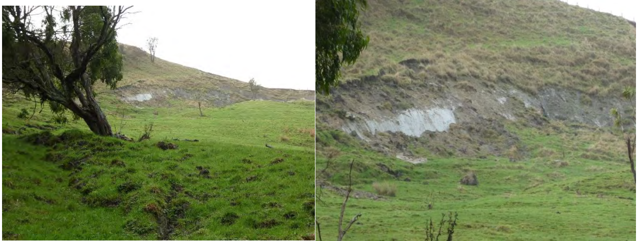
View of edge of landslide from above dam, toward headscarp
