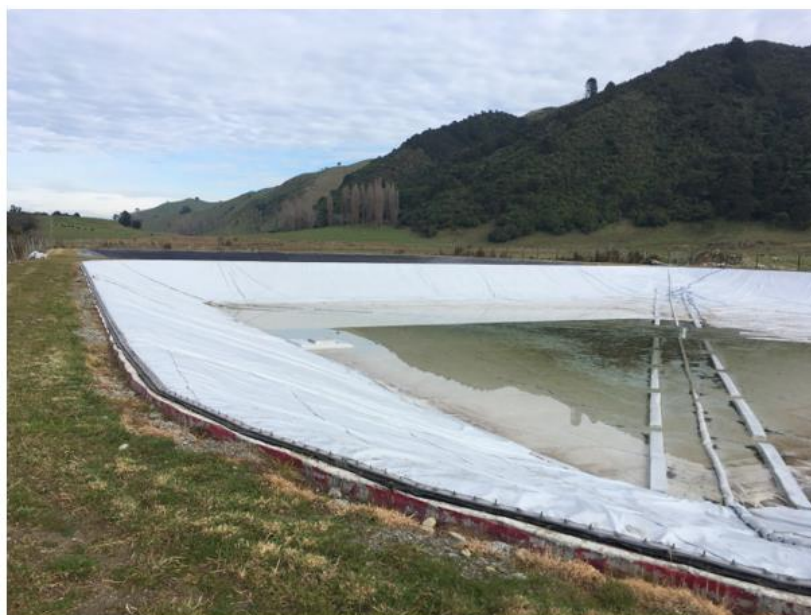
Figure 1. 8000m3 treated water storage at Waiohine treatment plant, ready for commissioning
