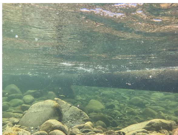
Figure 3 - Washout of rocks that supported the pipe
