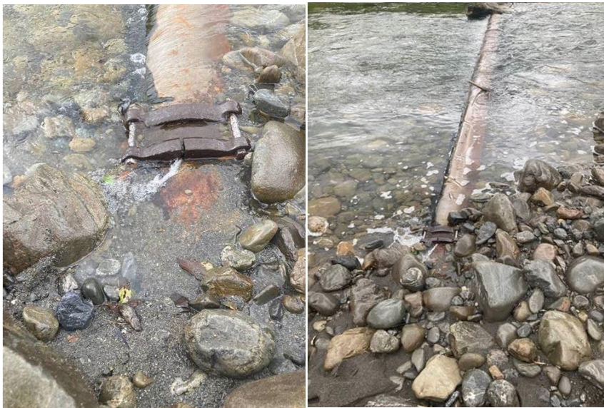
Figure 3. Coupling water leak on Featherston water pipeline within Tauherenikau River
