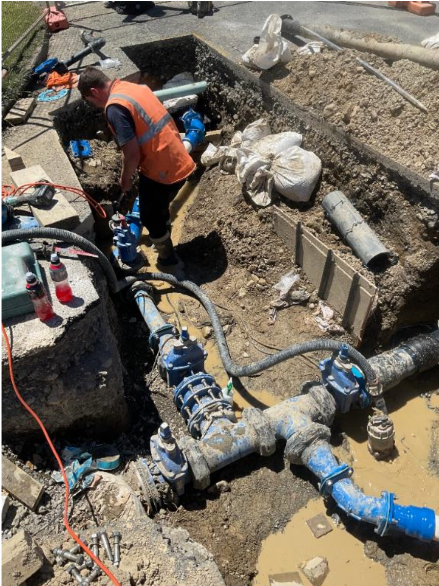
Figure 9. Contractors renewing the Fox Street water main, Featherston
