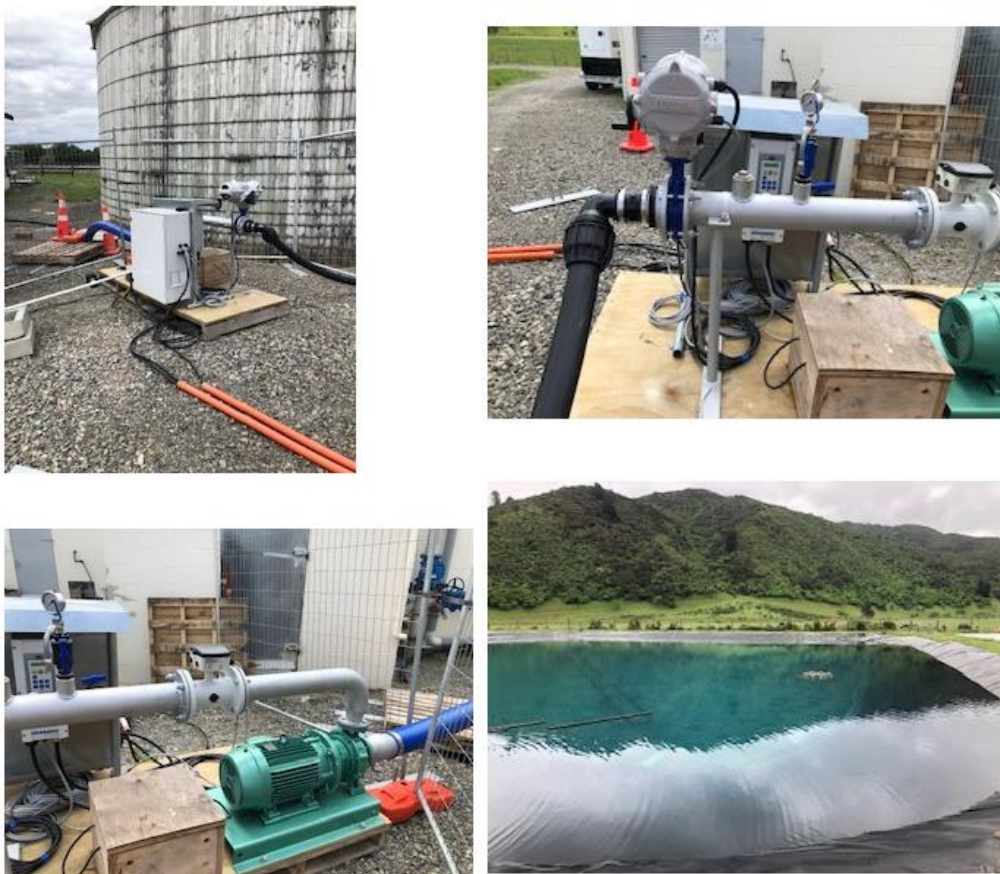
Figure 5. Recirculation pumping setup at Waiohine WTP for cleaning and disinfection
