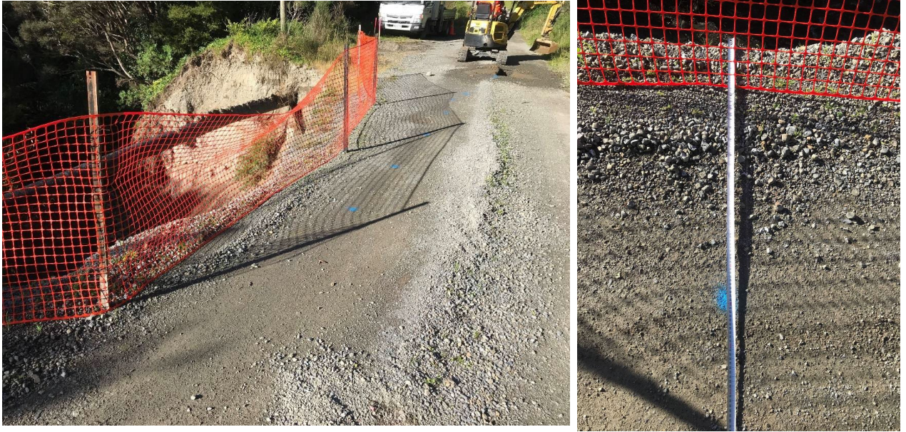
Figure 2 Boar Bush Gully Road slip, May potholing and water main location
