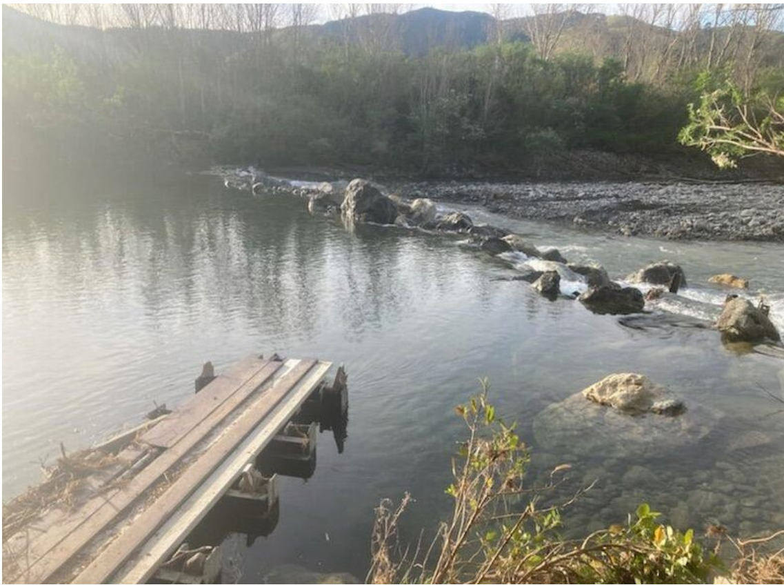
Figure 3 Longwood race intake rock weir being reinstated
