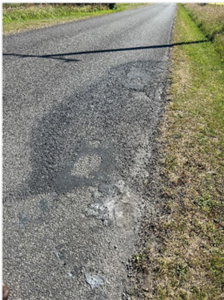
Image 19: Damage to road surface just past the bridge
