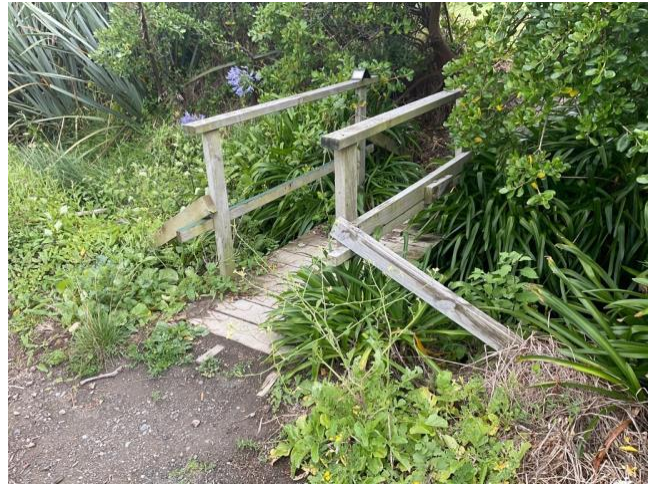
Site works - bridge
