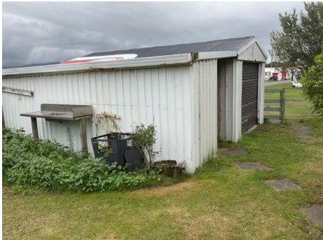
Garage 1 with storage
