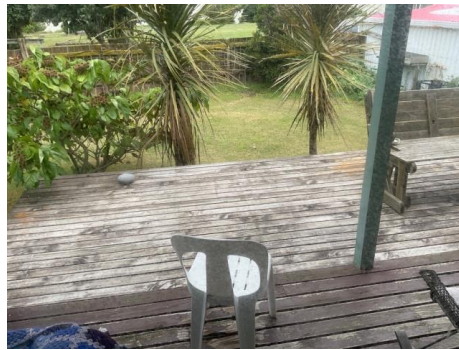
House - rear deck
