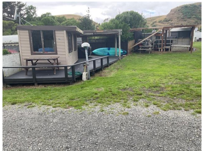
Site works - power
