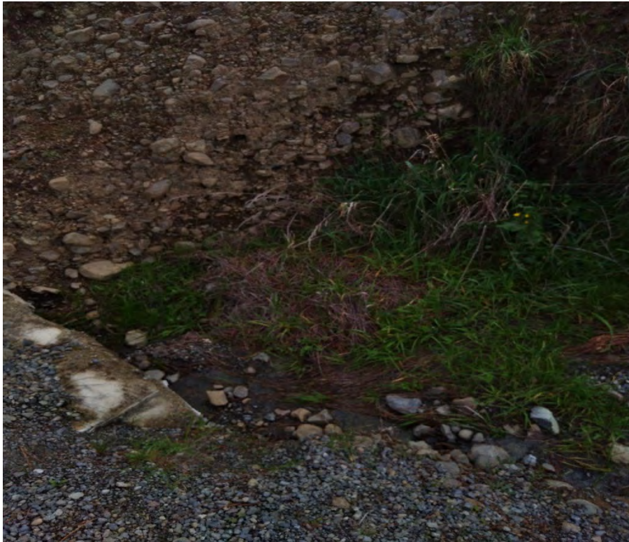
Figure 4 Blocked culvert
