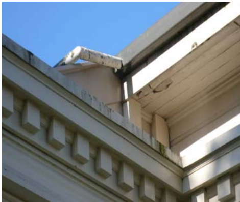
Soffit, with peeling paint indicative of leaking (downpipe needs paint.)
