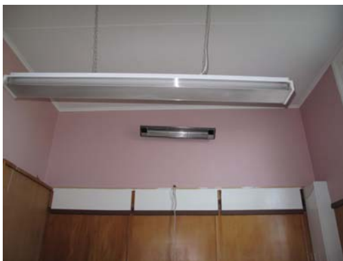
Office with fluorescent lights and heater. Wire hangs unfinished where a fitting has been removed.
