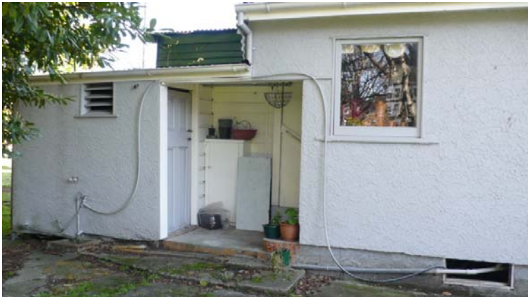
Back porch with nearly all the exterior maintenance items. Unpainted high level roof, untidy draped water piping, waste pipe, missing access door, old DP bracket.
