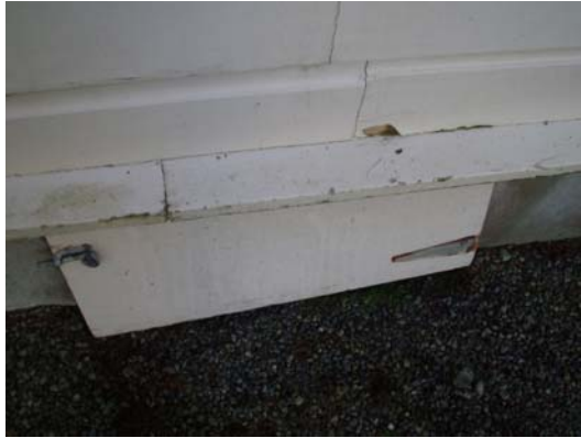
Sub-floor access door with broken hinge
