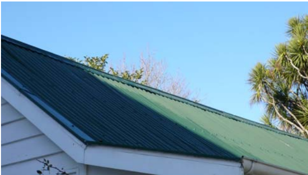
Roofing with some loose ridging
