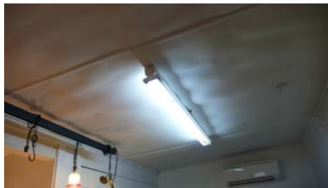
Battened modern sheet linings, fluorescent light and AC unit are all out of place.
