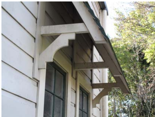
Detailing to south wall window hood
