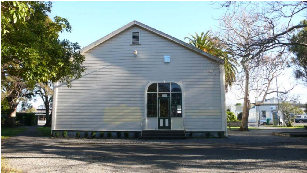
East wall with added door in glazed frame (this element is central in the ‘big room’). (The modern extract fan is an intrusive item)
