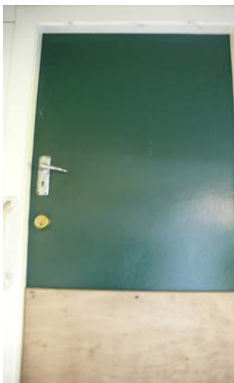
Back door. Non-original modern flush door with patch, presumably over damage.
