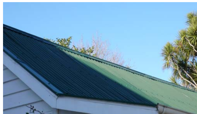
Roofing with some loose ridging.
