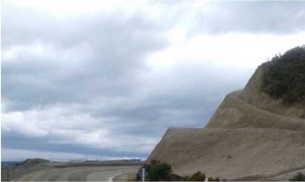
Whatarangi Cliffs: Benching and Road construction work
