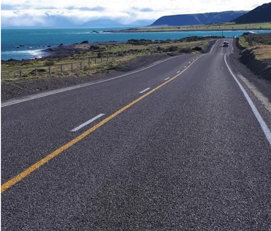
Cape Palliser Rd seal extension
