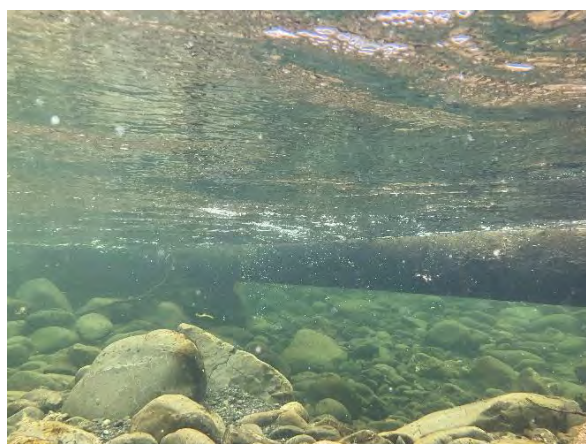
Figure 3 - Washout of rocks that supported the pipe
