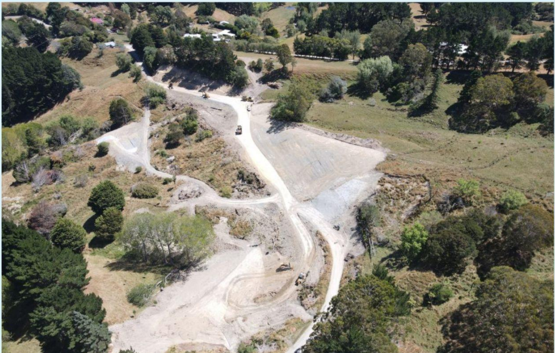
Hinekura Road remediation, February 2024.
