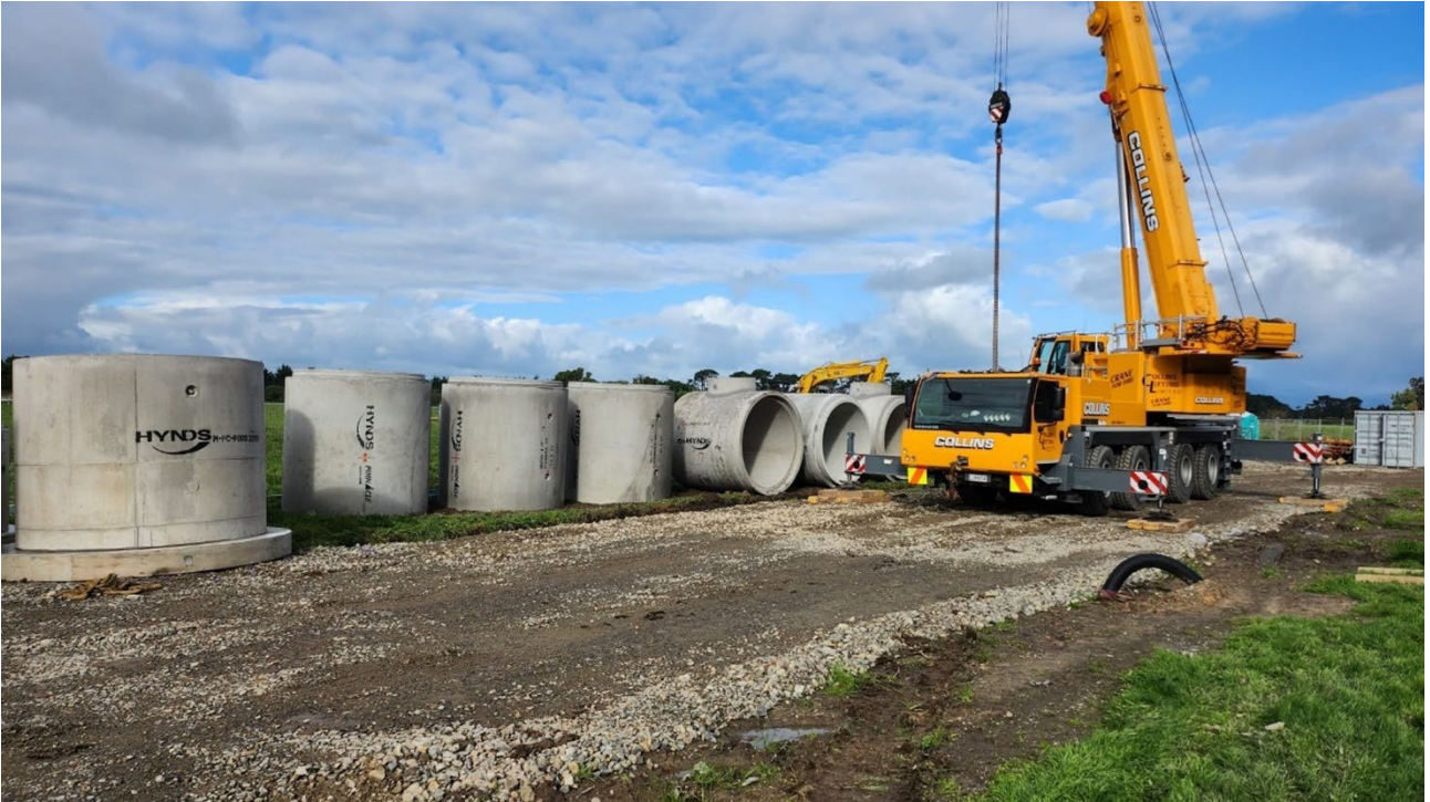
Upgrade underway on Featherston's Donald Street wastewater plant
