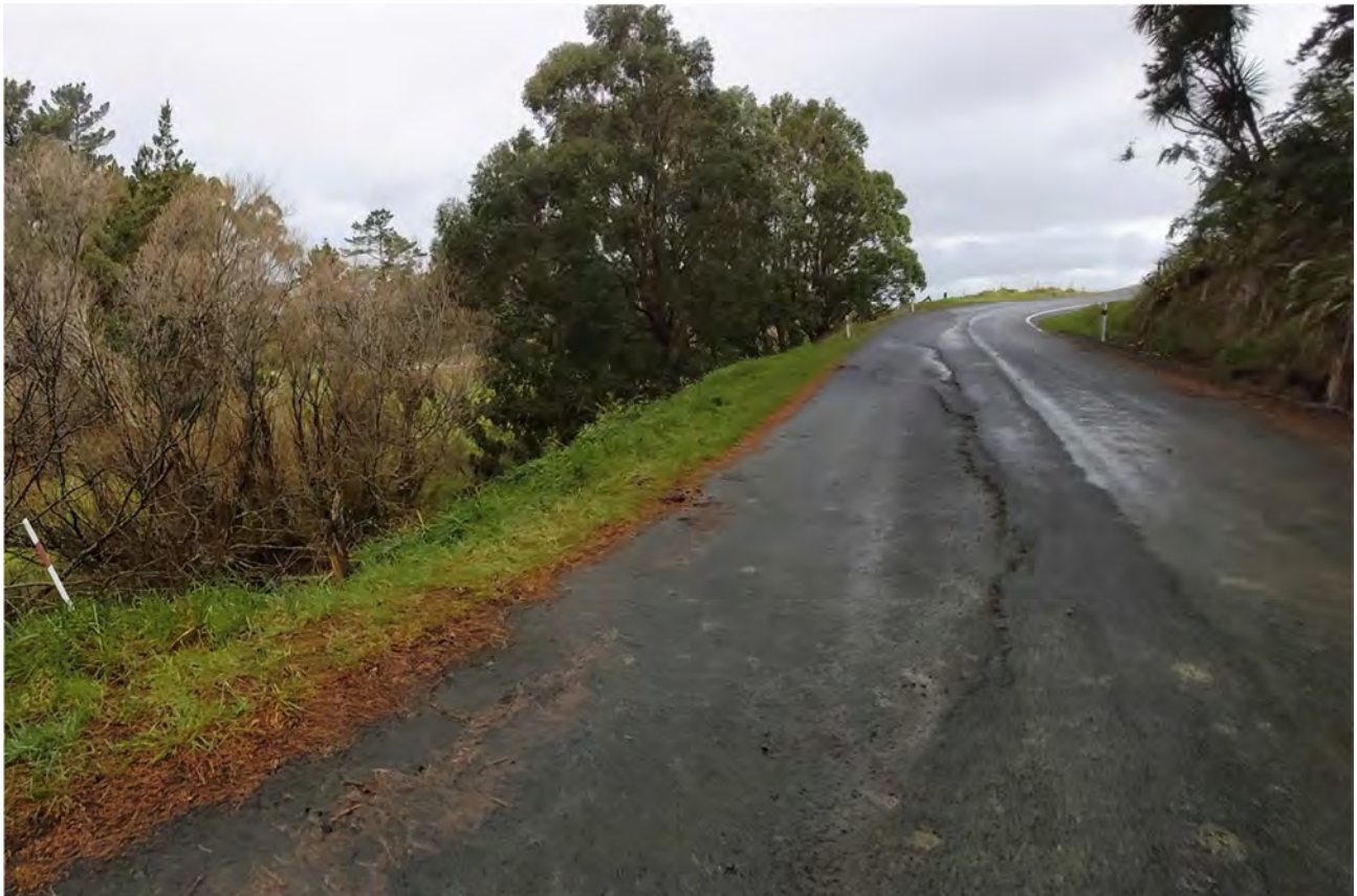
Figure 4: Developing underslip on Hinekura Road immediately upslope of southern farm dam, about 400m east of the main landslide
