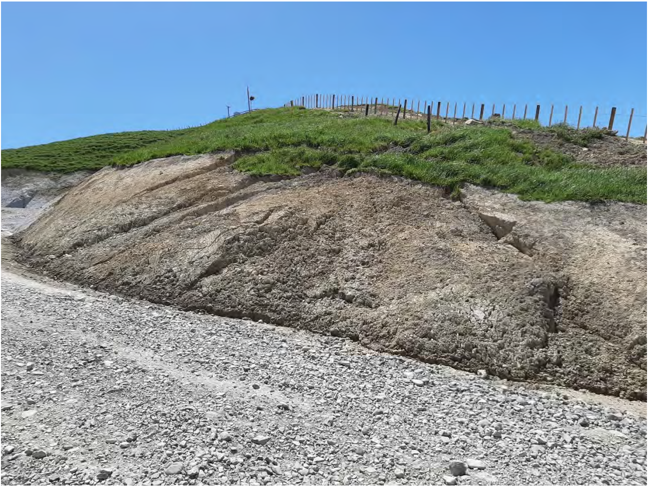
Figure 22: Moderate sized overslip developing above recent temporary road
