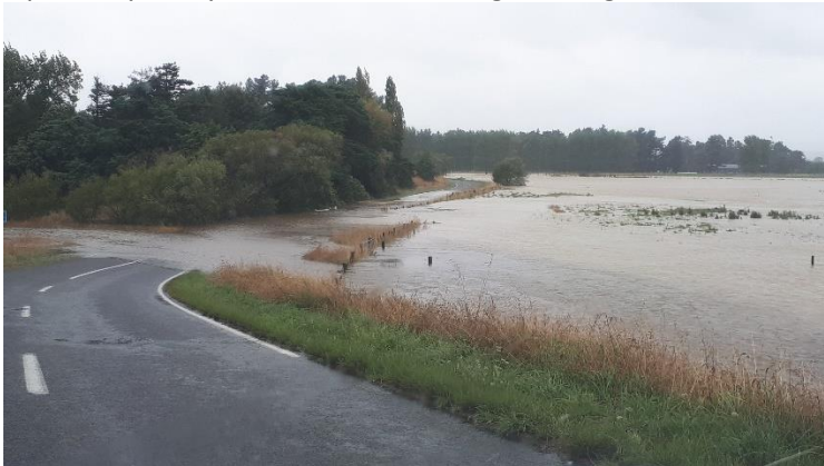
Pahautea Rd Spillway working as designed
