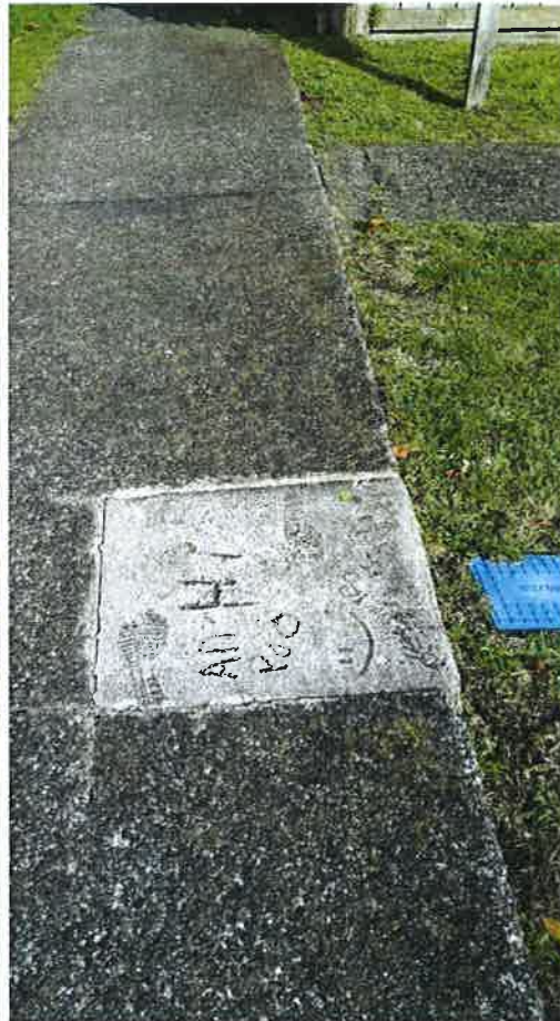
Repair with uneven surface
