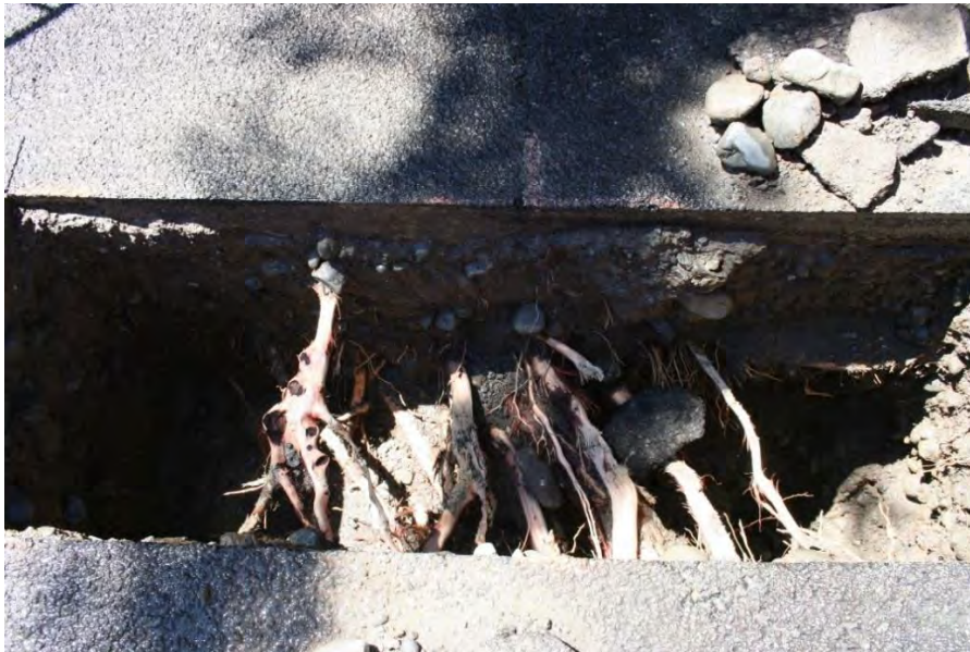
Fig.A1.10 A mass of roots where unearthed 20 cm-50cm below the surface. Largest root measured 15cm in diameter.
