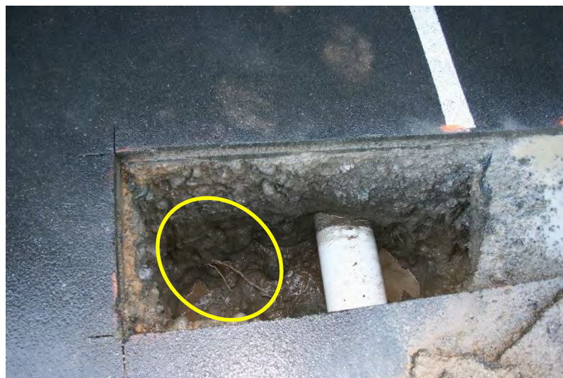
Fig.A1.9 Hydro excavation was carried out to the desired depth. Only two minor roots were unearthed (highlighted in yellow).
