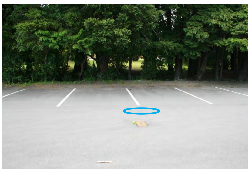
Fig.A1.7 Pothole 2 located further along the alignment. Adjacent to totara and Lawson cypress, roots rarely occupy the same area so pot holing at this location is a good test as the trees are more closely grouped.
