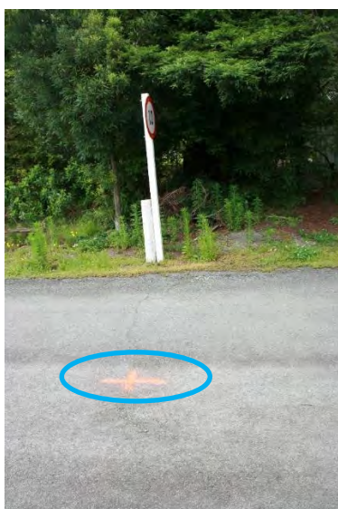
Fig.A1.6 Pot hole 1 Located over the area that shows potential root conflict (root spread from redwood (shallow rooted species note cracking of pavement))
