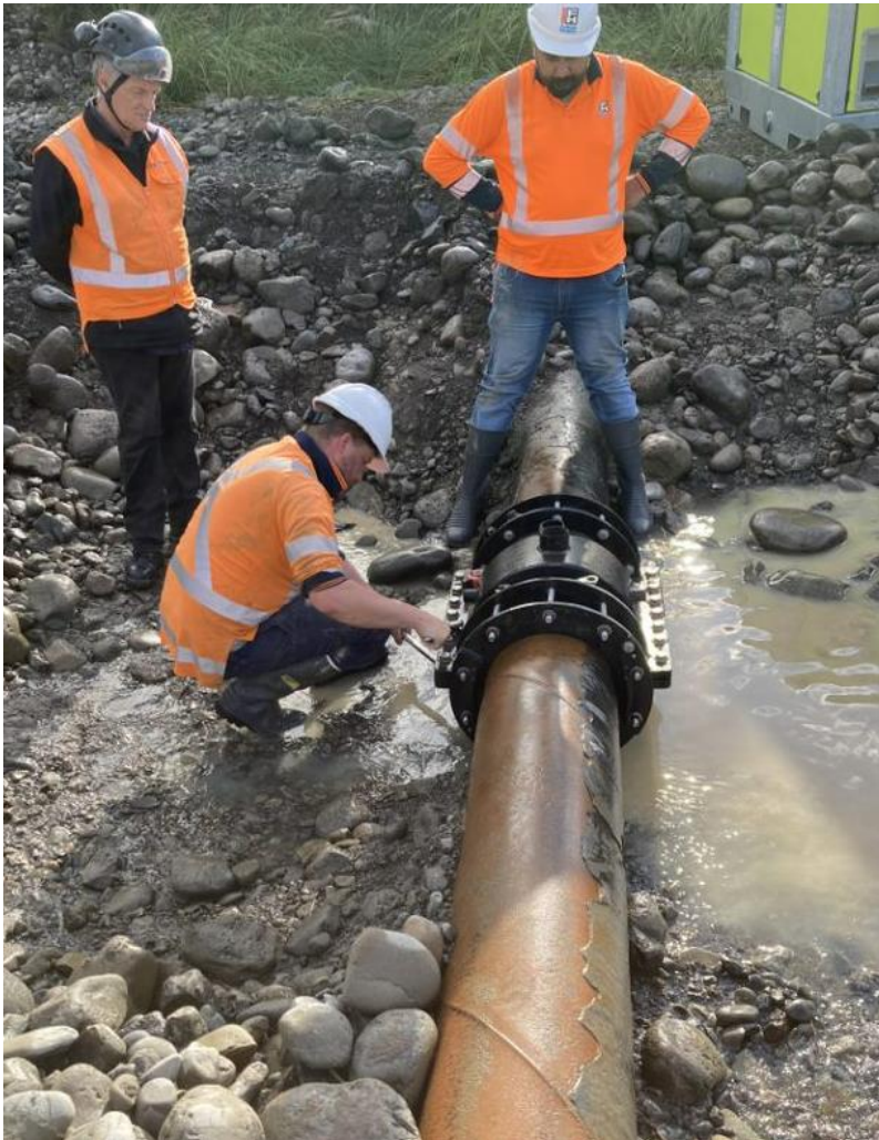
Figure 3. Clamp being installed at the site of the leaking joint, Tauherenikau river
