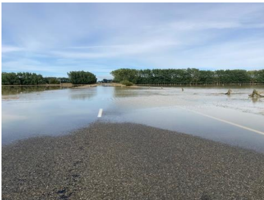
Oporua Spillway Kahutara Rd working as designed
