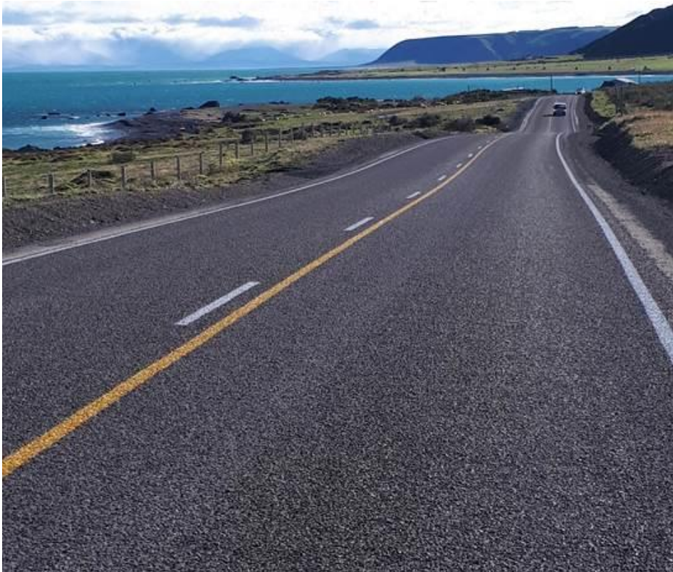
Cape Palliser Rd seal extension
