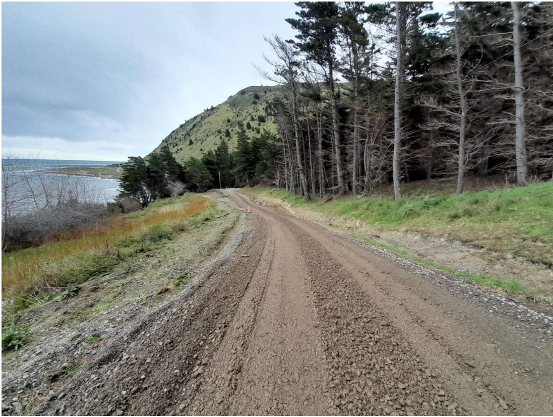
Newly graded filled section
