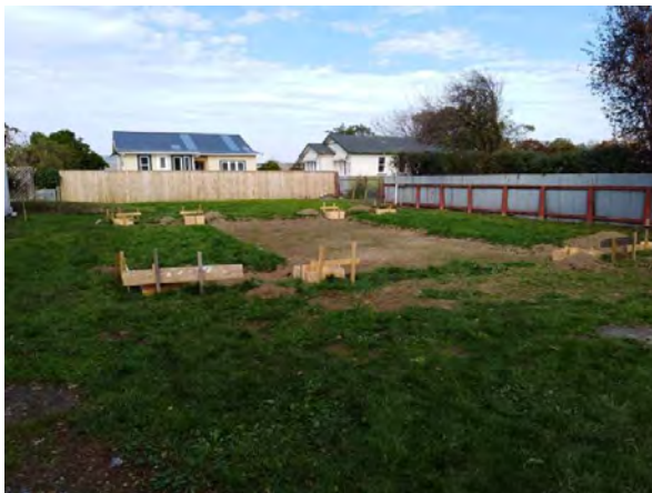
Measuring out boxing for container pads 8/5/19
