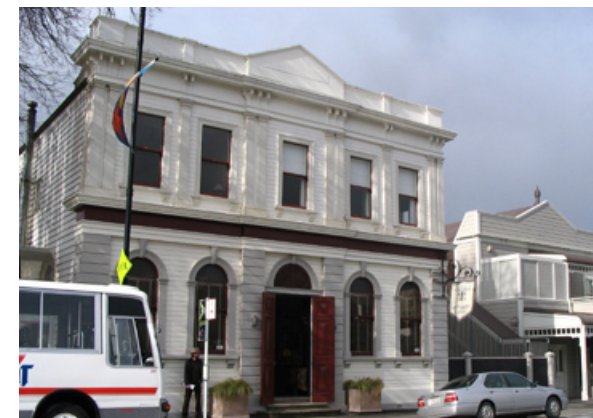
The expression of floors (through horizontal modulations) scales this two storey building to the street. The pilasters and windows provide vertical modulation creating rhythm.
