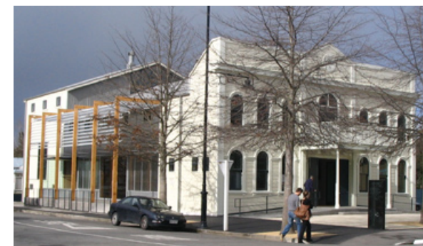
The renovation to the town hall, while contemporary in form, manages to pick up on the rhythm of verandah posts that typify the town centre. This approach is preferred to a simple mimicry of the facade in a new addition.
