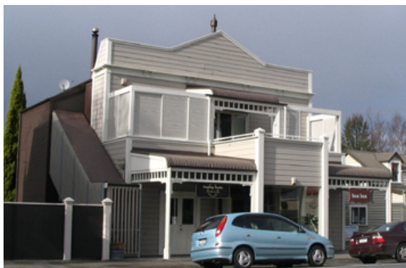
Alterations using materials and colours which are in keeping with the original building.
