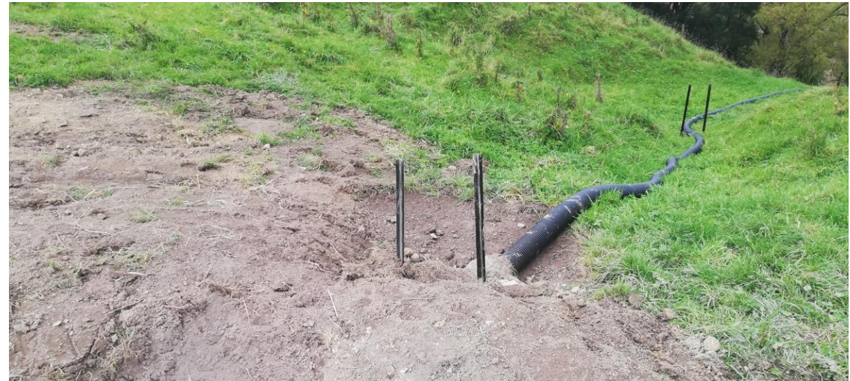
Novacoil going from the lowest V drain towards the culverts on the eastern side of the slip
