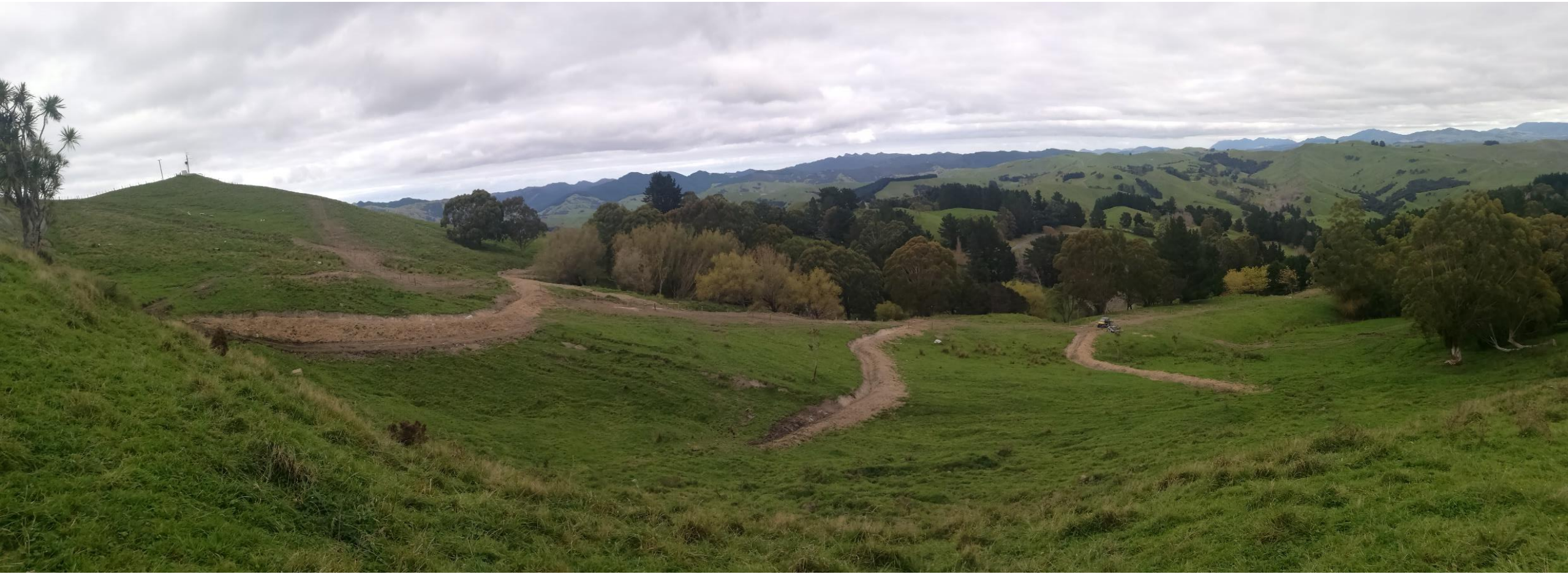
Panoramic view of the topside of the slip. With the 3 V drains and fence
