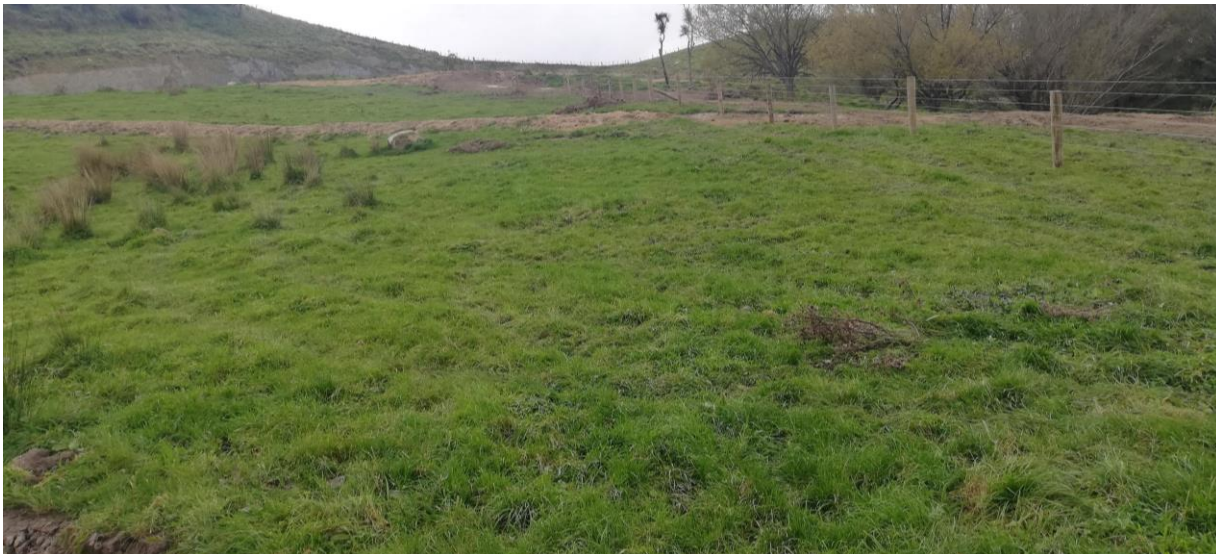
New fence on upper side looking up. Can see the 'cliff face' of the slip in the background
