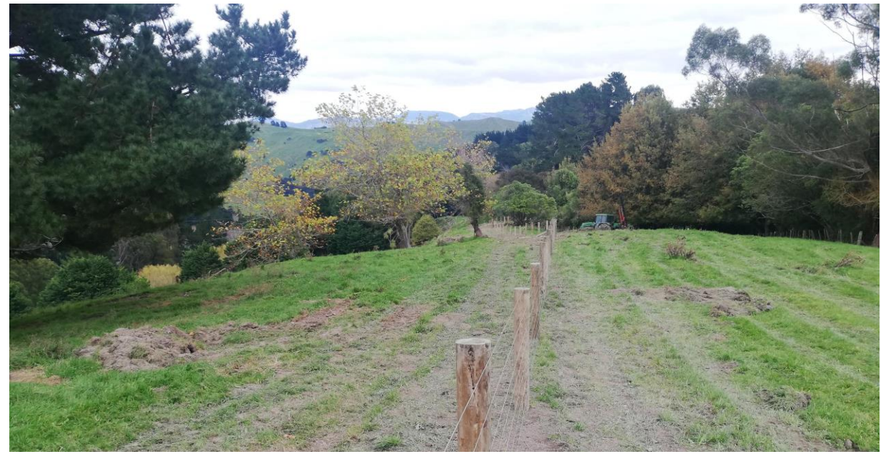
New fence looking to the east side of the dam
