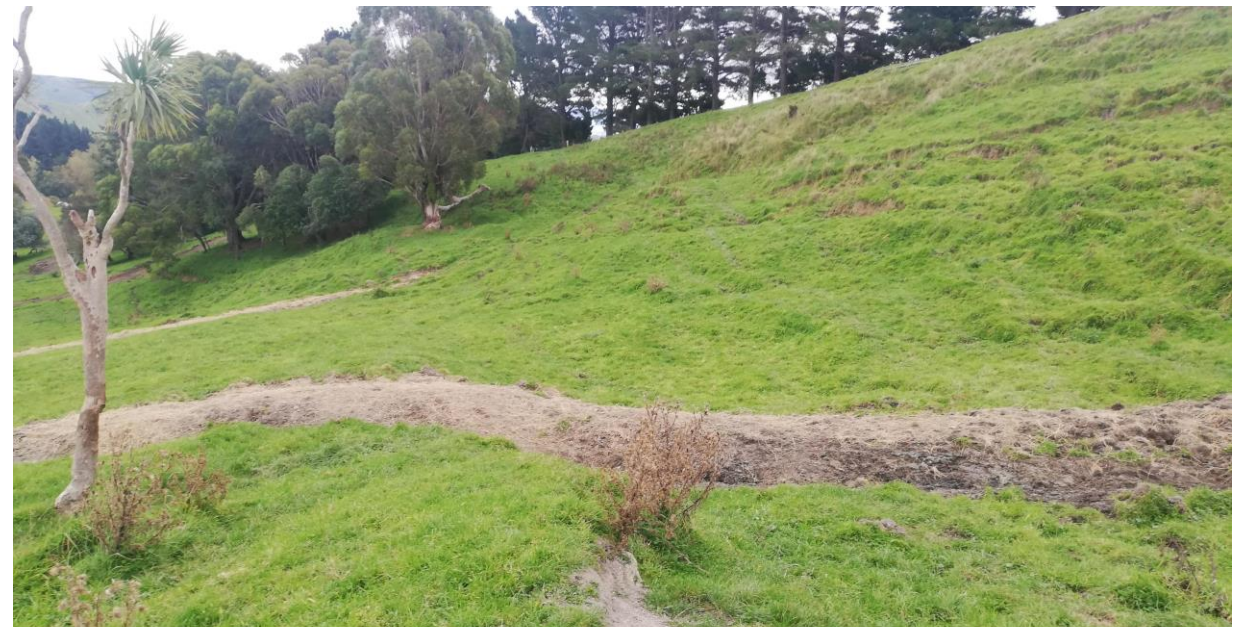
Looking at the slumping at the western side of the slip at the top
