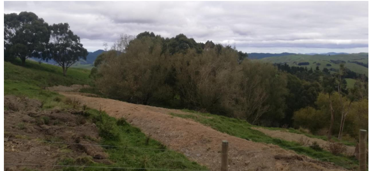
New fence and 1 of the V drains looking east
