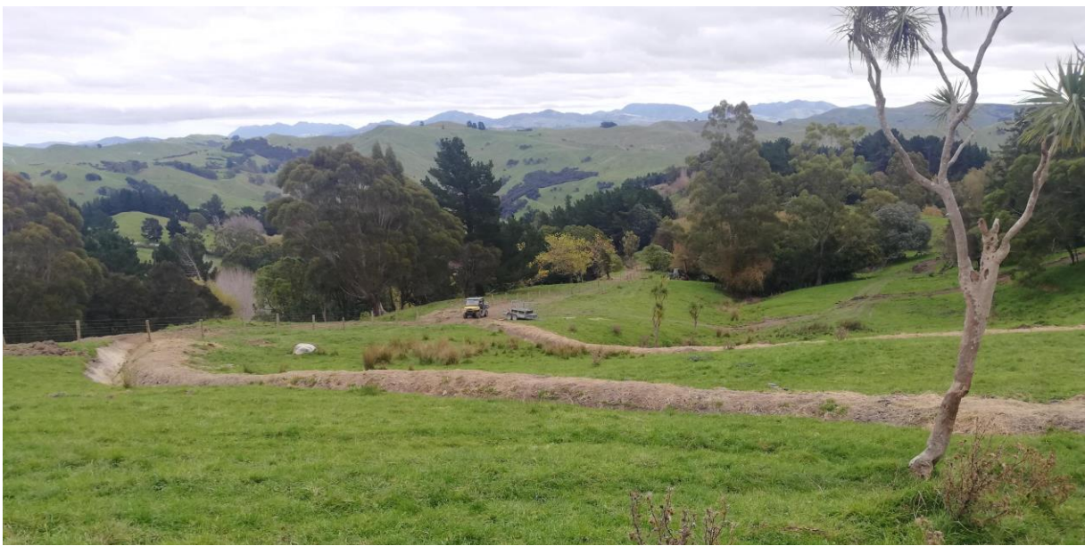
New fence and 2 of the V drains looking down hill
