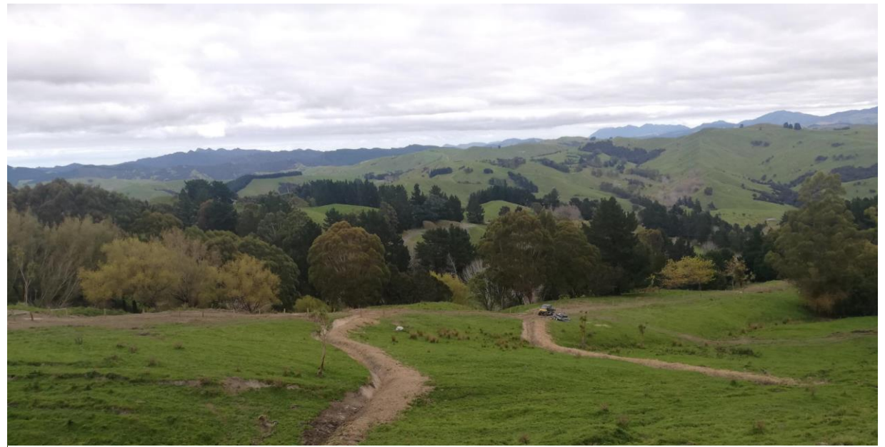
New fence and 2 lower V drains looking down the hill
