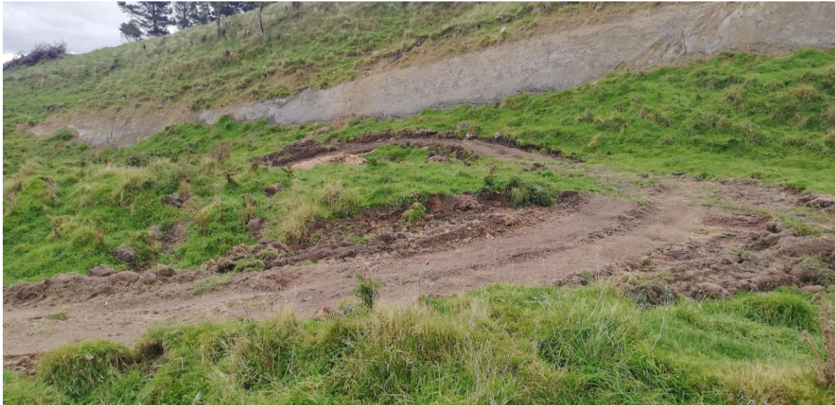
The 'cliff face' at the top of the slip
