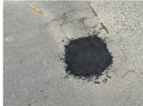
Pothole repaired
