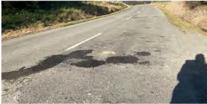
Pothole repaired on Hinakura Road
