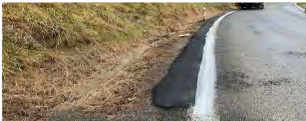
Edge break repairs on Martinborough/Masterton Rd
