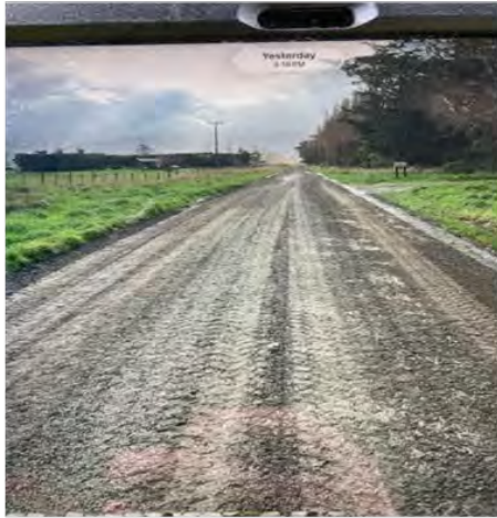
Unsealed road grading and metalling on Kumenga Road
