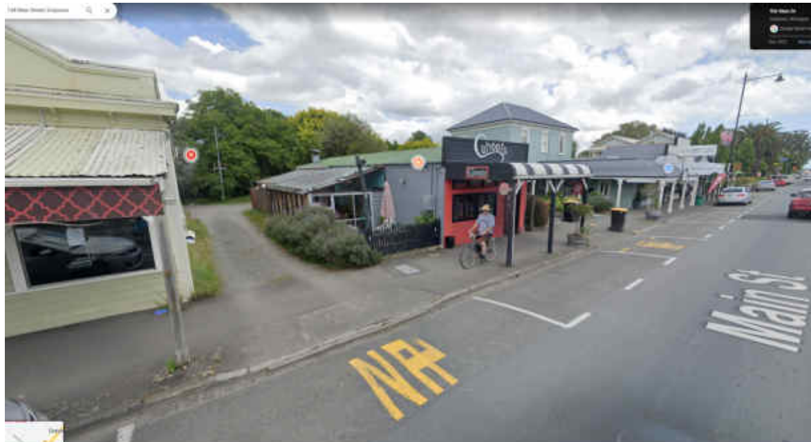
Figure 8- kerb crossing example at Cahoots Café 97 Main Street, Greytown, 3.5m wide with partial apron at the kerb and footpath running through behind. Source, google maps December 2022
